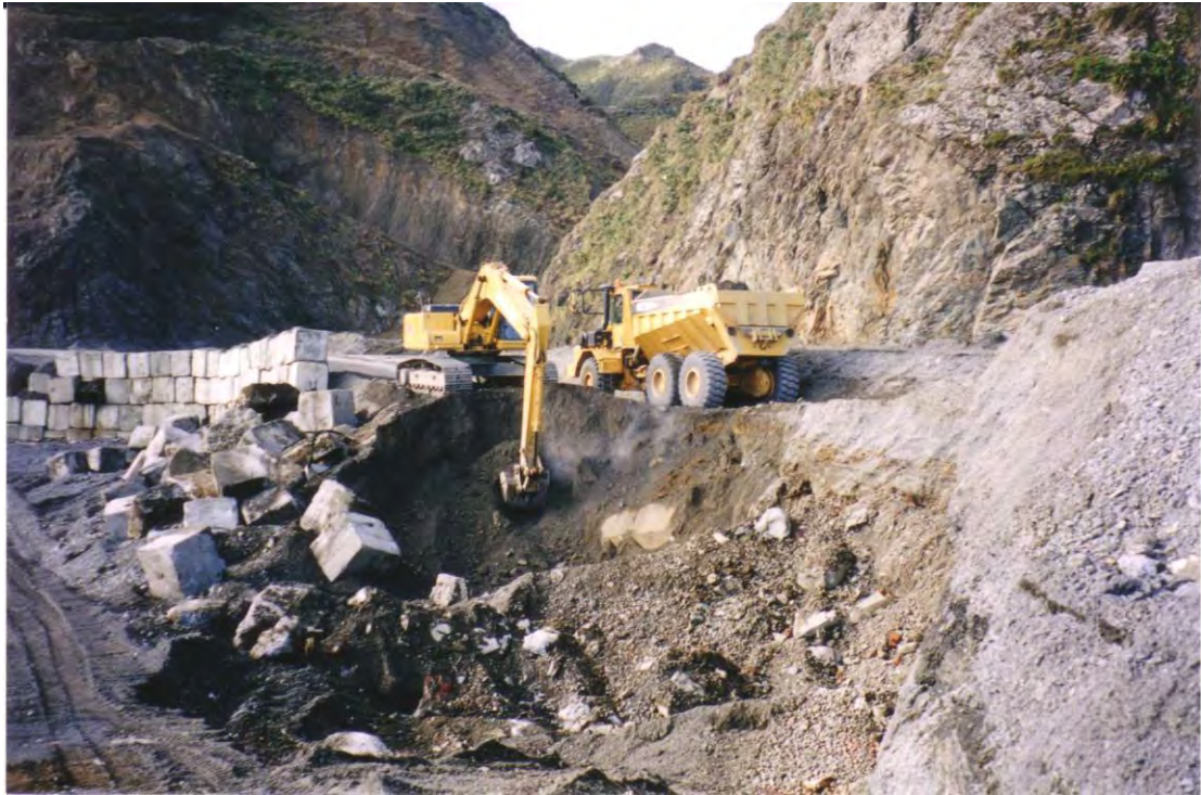
Earthworks on Hape stream area get underway.
