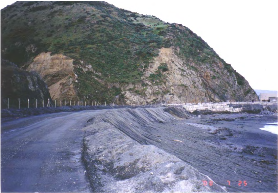
Hape stream area prior to rehabilitation work.
