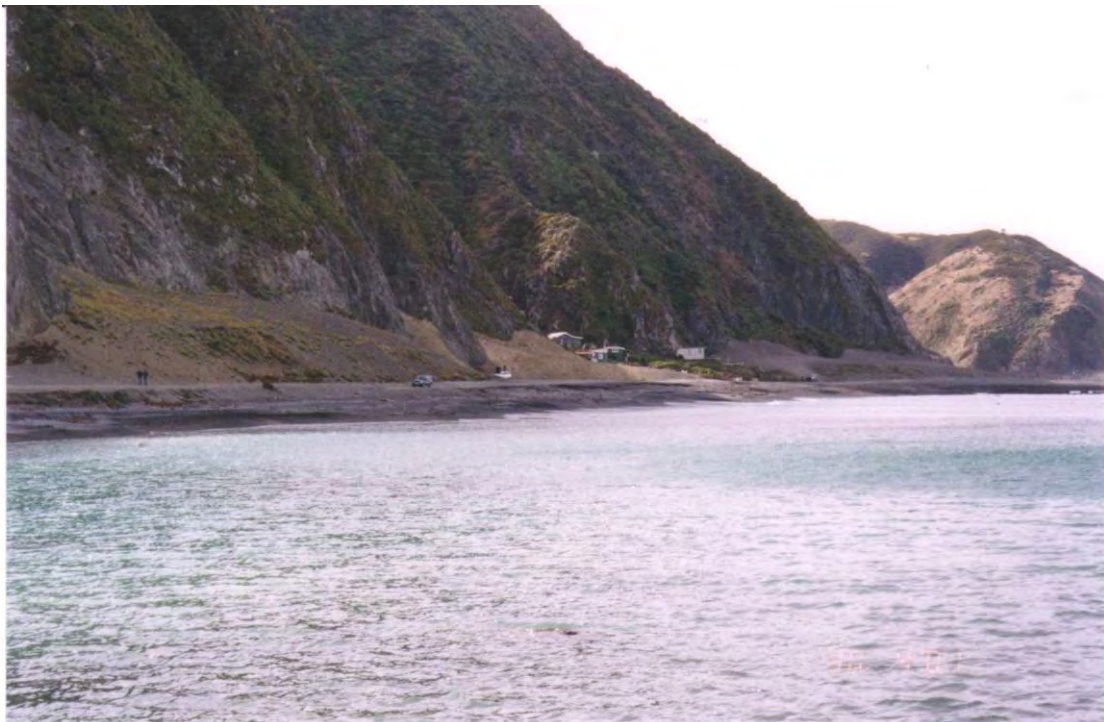
Sea view of another completed area.
