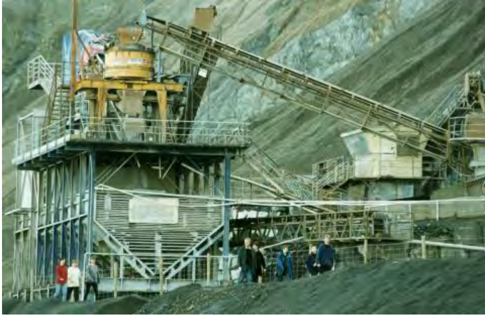
Members of the public walking past the quarry crushing plant.
