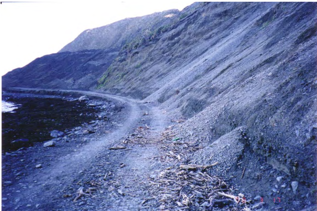
Coastal road. This area required special attention to ensure that following re-shaping, wave and tidal action did not result in silt being washed into the sea.
