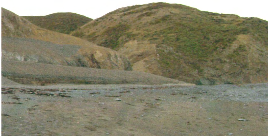
Hape stream following re-shaping.
