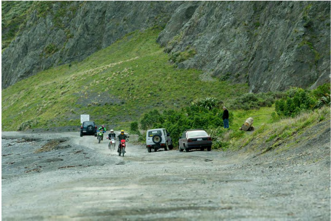
Planted area in background. The toe of the batter (slope) was shaped to try and prevent vehicle damage.
