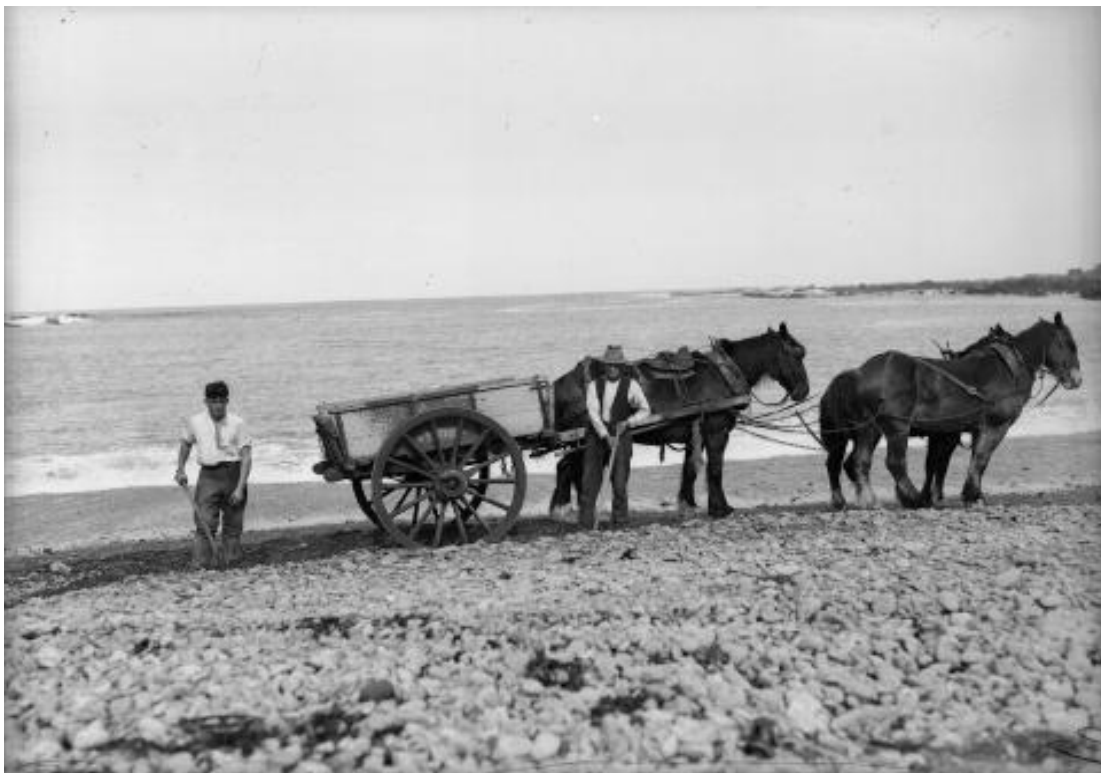
Employees of Tonks and Andrews collecting shingle from Owhiro Bay.
