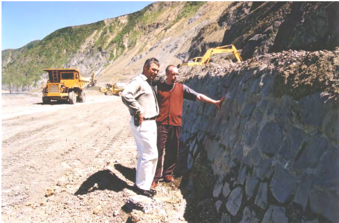
Wellington City Council staff check out the newly exposed sea wall.
