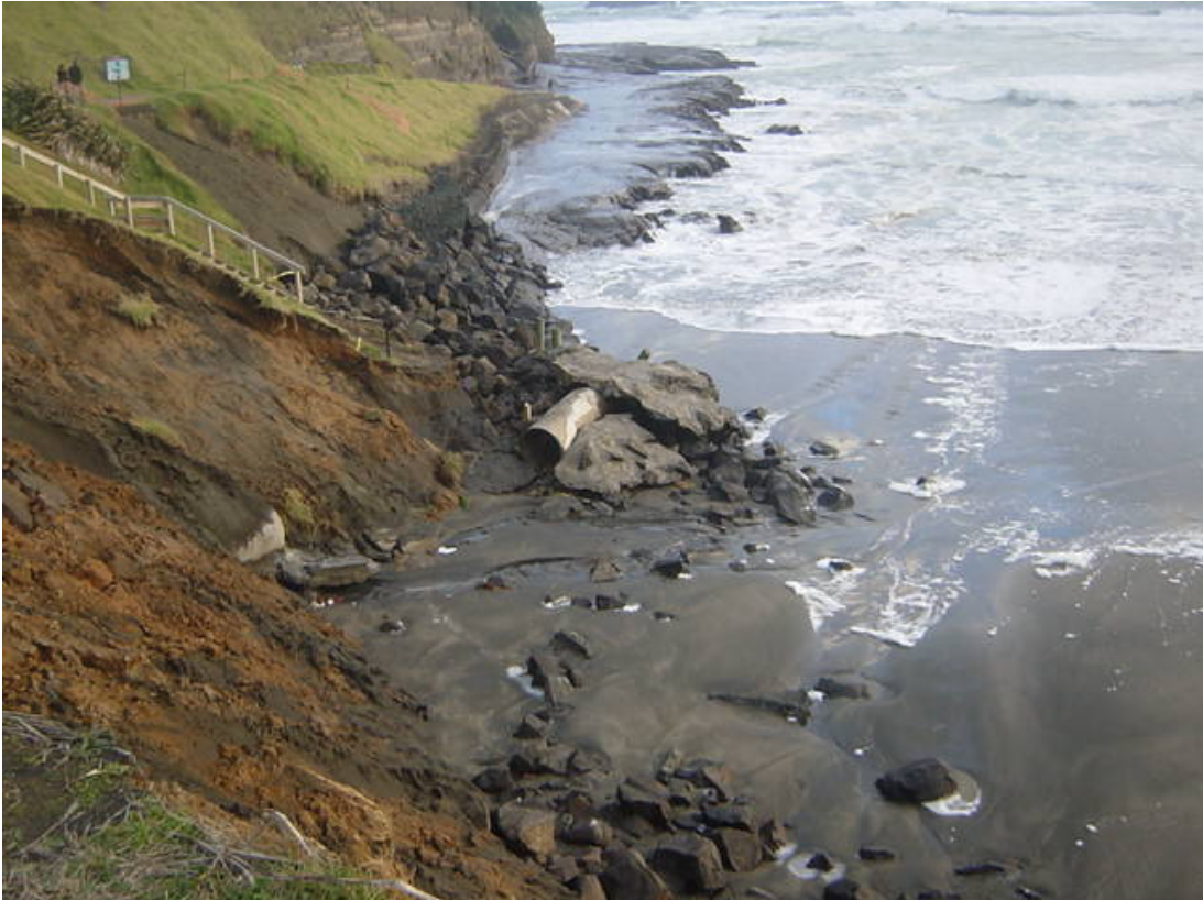
Figure 1: Erosion at Muriwai Beach, west of Auckland (Source: PHILLIPS, 2006)
