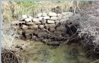
Flapgate and channelisation in Okiwa Bay.
