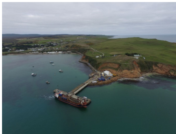
Figure 3 – The existing wharf at Waitangi showing the T-shaped wharf and small operational area.
