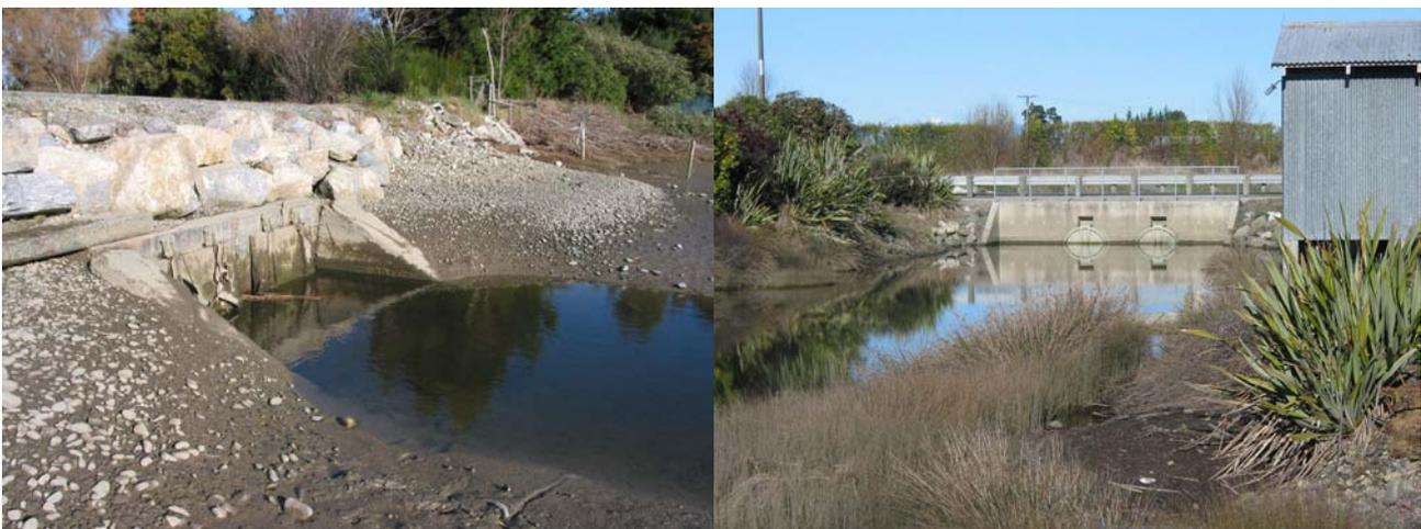
**Figure 7.** Flap-gates such as these effectively exclude migratory freshwater fish from reaching habitat above these structures.
