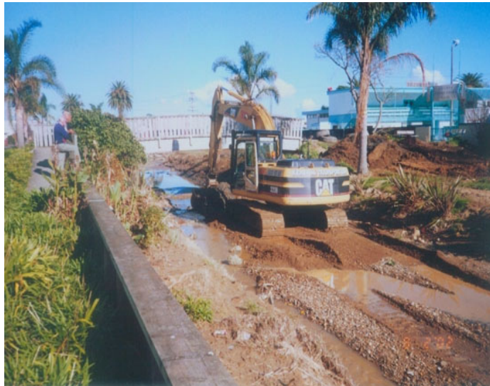
Figure 5: Clean up works in progress on the Hape Stream in Thames.
