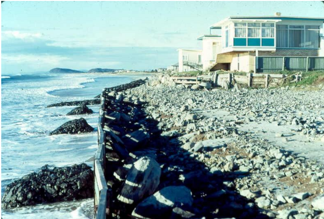
Figure 1.1: Severe erosion at northern Waihi Beach in 1974. Photograph taken by T.R. HEALY (1974).
