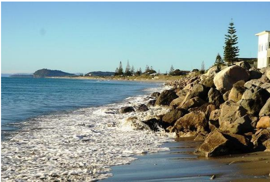
Figure 1.2: The seawall in its present state at Waihi Beach showing the lack of beach at high tide. Photograph taken by the author 28/05/08.
