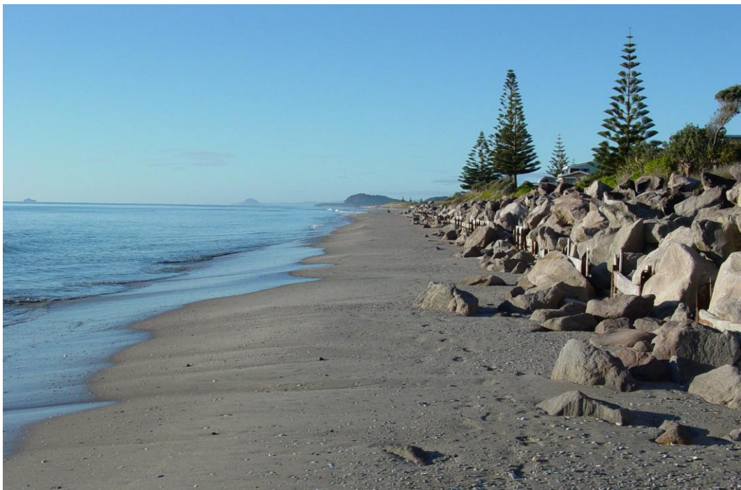
Figure 3.4: The rock revetment at CCS50, which is located midway along The Loop. Also note the remnants of the older timber wall. Photograph taken by the author 24/06/08.
