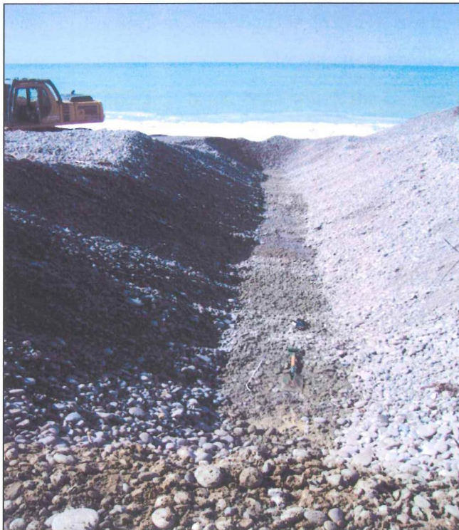
Figure 5.8: Photo of the trench site at McLeays Road (S6885).
