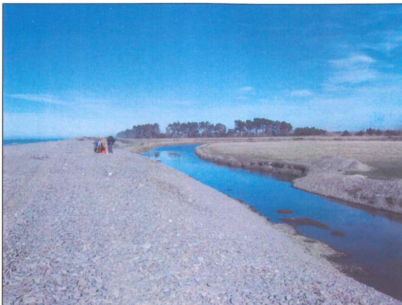
Figure 5.1: The Waimate creek site (S5554), displaying the Waihao Dead Arm to the backshore of the barrier.
