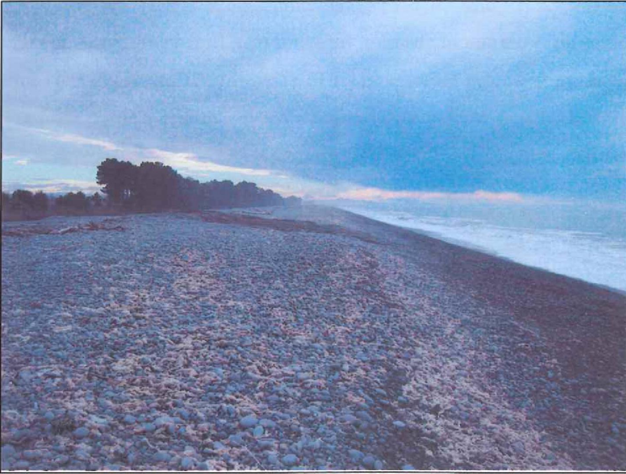
Figure 1.3: Photo of the Waihao-Wainono barrier at the Lows Road site.
