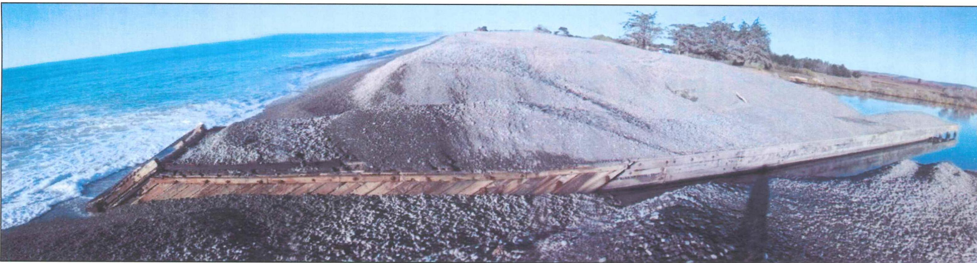
Figure 3.5: Photo of the Waihao Box Outlet. The sea is to the left and the Waihao River is to the right of the barrier.
