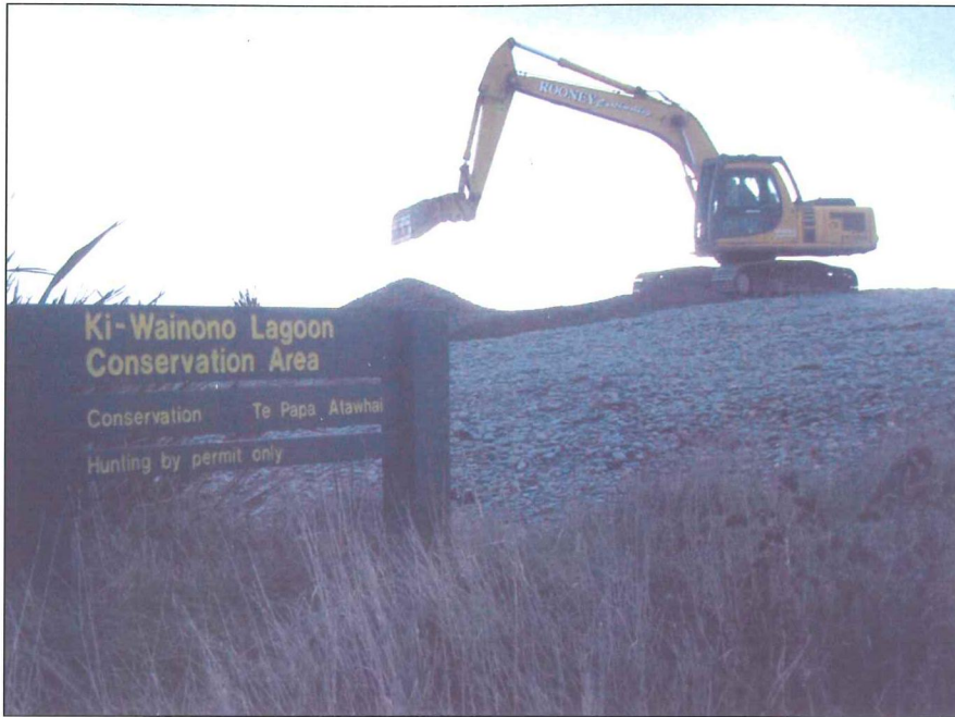
Figure 5.11: Photo of the Lagoon area. Site is Wainono South bank (S5320).
