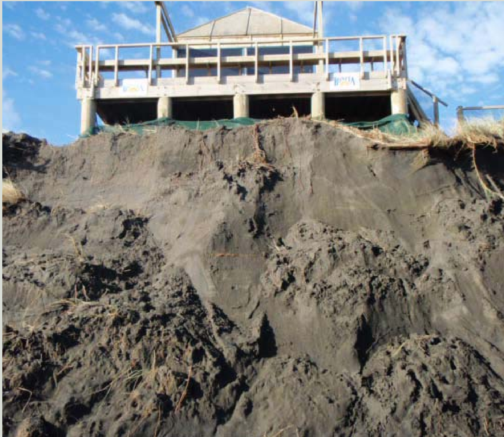
Old Muriwai surf life saving tower after dune erosion
