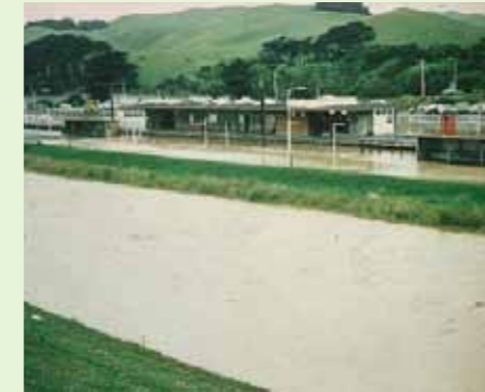
Past flooding at Porirua Railway Station, 1976.
