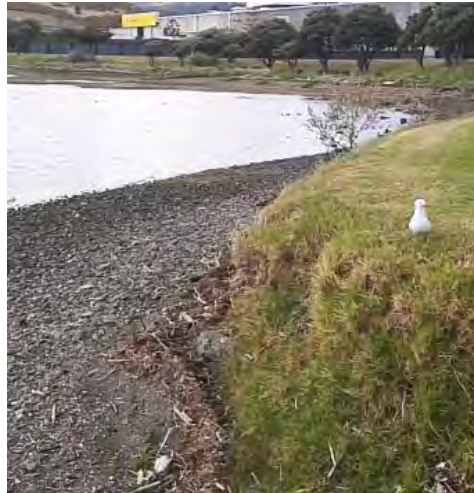
Reclamation material eroded by wave action creates a barrier to water access
