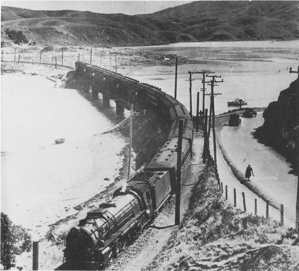
Fig. 9 – Paremata railway bridge in about 1930. A line at the foot of the hills follows the present Camborne Walk. Note the absence of any settlement north of the bridge. (Photo courtesy of Porirua Museum.)
