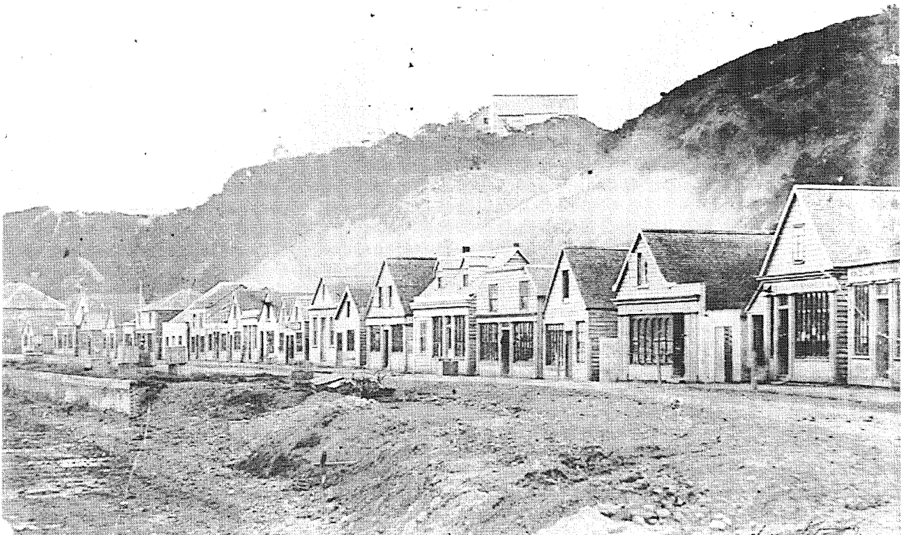
Fig 43 a. Post-earthquake (1860) photograph of Lambton Quay. Typical wooden houses are shown together with the fill (earthquake debris?) behind the uncompleted sea wall that was presumably abandoned after uplift made it unnecessary. The cutting shown in the central part of the photo is the location of the present cable car (Ref. No. B3926-1/2, Alexander Turnbull Library, NLNZ).
