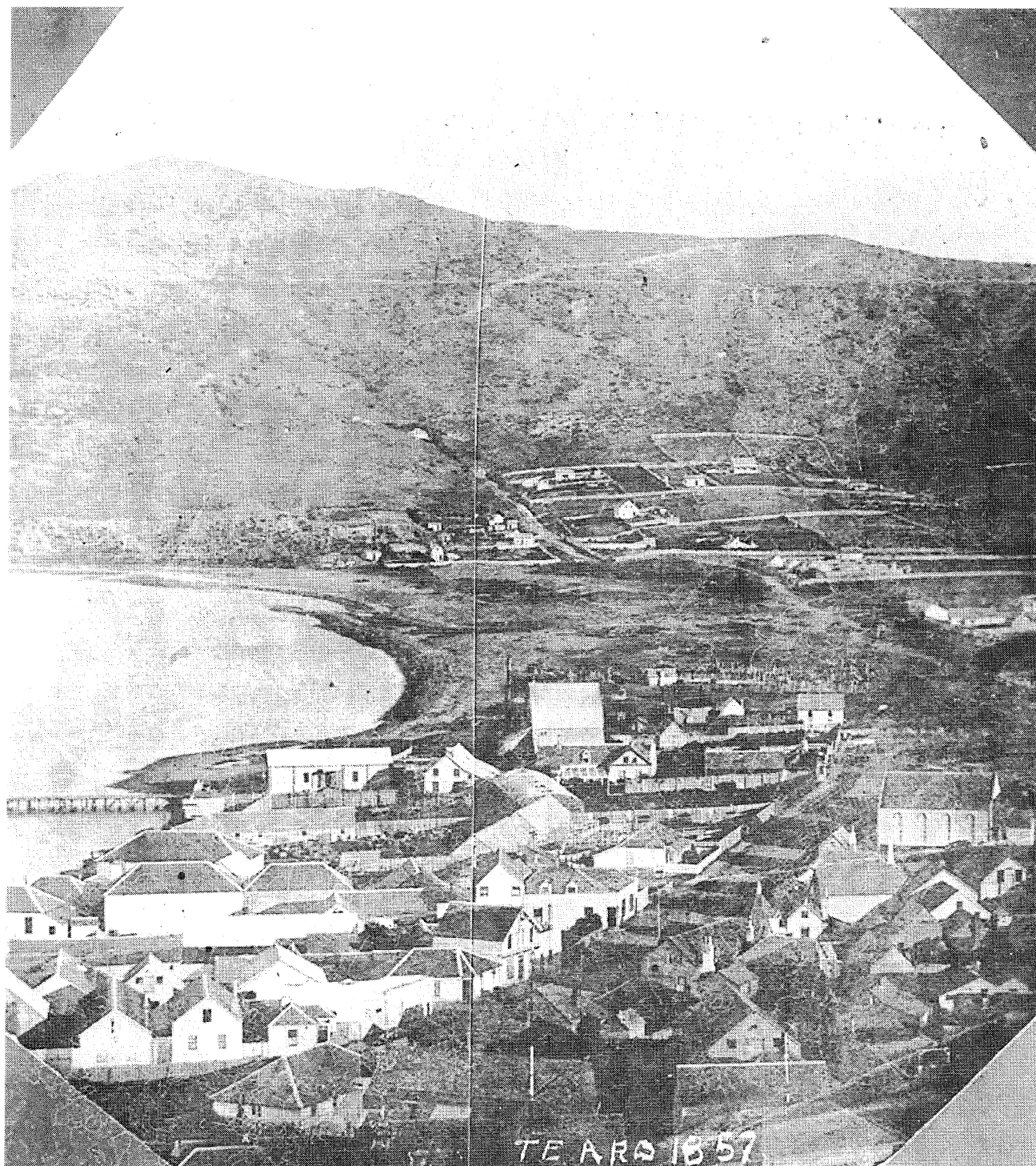
Fig.18. Photograph by F. J. Denton (c.1857) looking east towards Mt. Victoria and the Te Aro foreshore, Wellington, and showing the widened area of beach exposed by about 1.5m of uplift during the 1855 earthquake. The post-1855 high tide mark can clearly be seen (see text). (Ref. No. F145534 1 / 2 , Alexander Turnbull Library, NLNZ).
