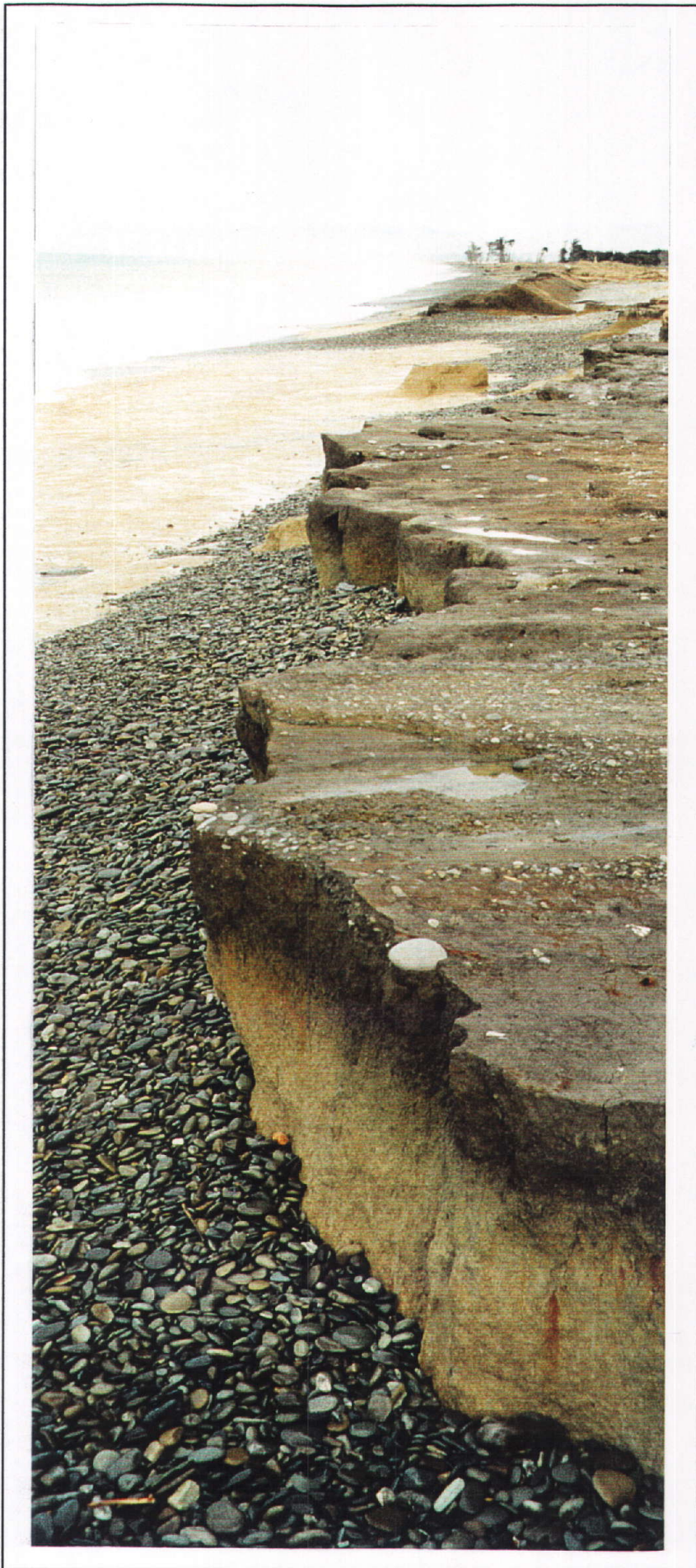
Figure 6.1 Significant Erosion of Old Coastal Stopbank at Connolly's Rd.
