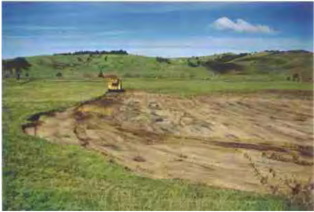
Figure 7. Preliminary earthworks in NU 4
