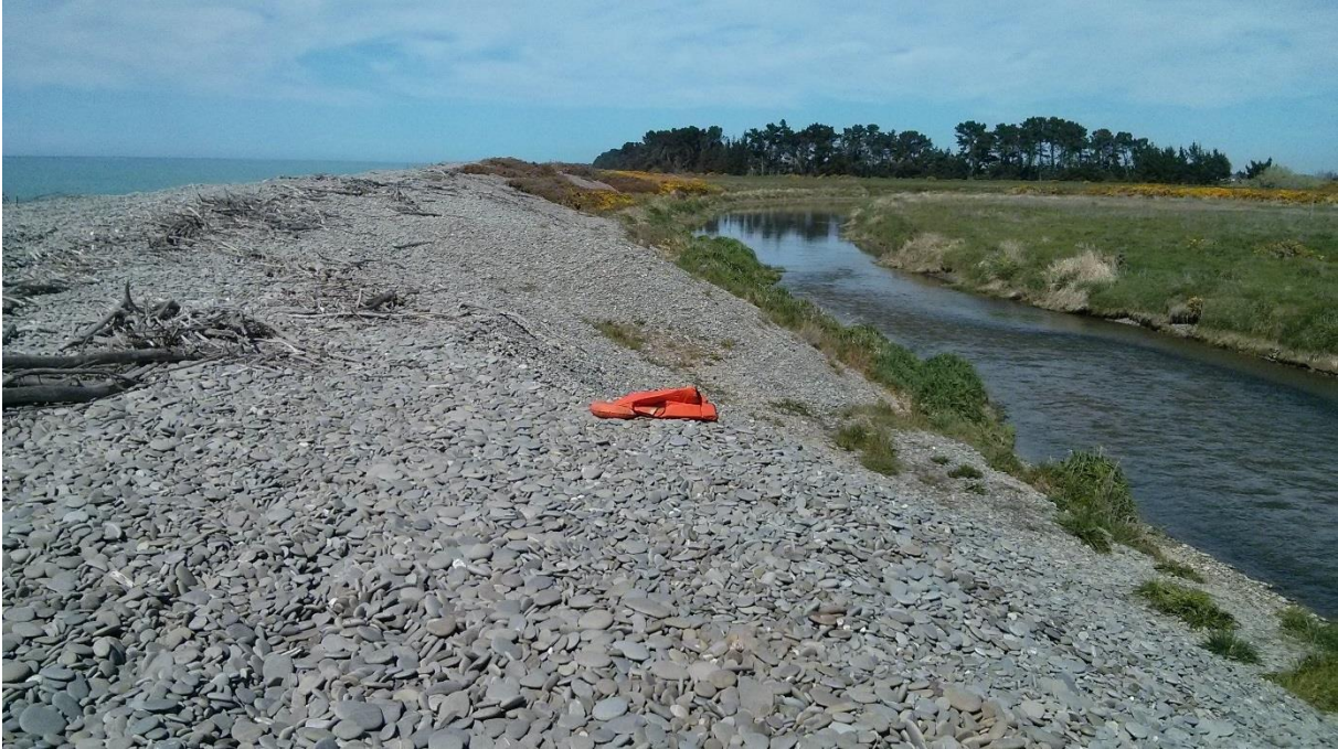
Figure 4-5: View south along barrier and old Waihao Arm channel at proposed outfall site. Note driftwood line showing extent of relatively recent wave overwash, steep backshore slope, and gravel riffle in channel formed in breach deposits. Near-field crest elevation is 5.5 m, rising to 7.0 m in distance.
