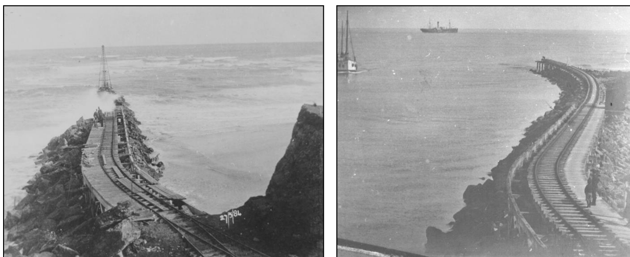
Figure 4 Construction of the original North Mole underway in 1884 on left, and the final structure curving into the prevailing wave direction several years later on the right. Note the beach accretion against the northern (right hand) side of the mole.
