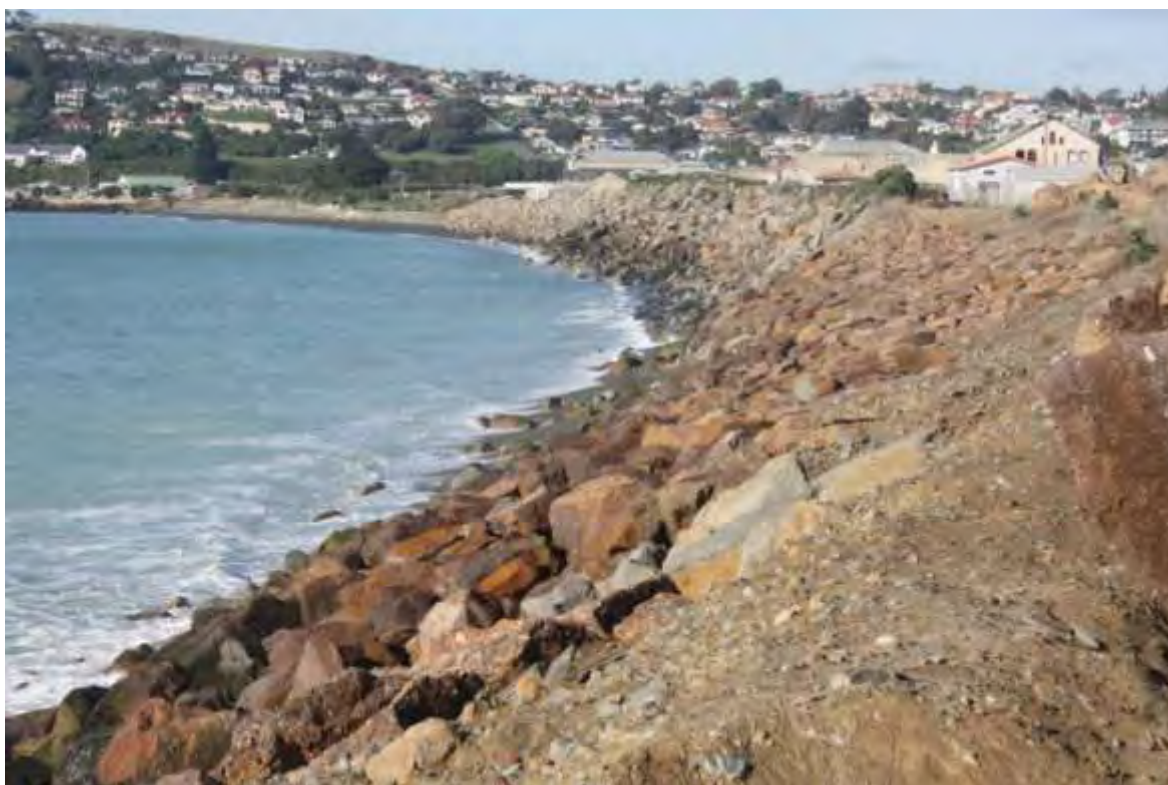
Figure 9-7 Rock revetment at Oamaru
