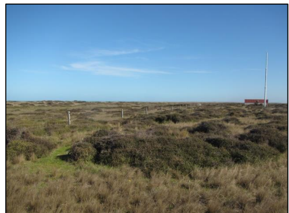
Plate 6: Southern boundary of the Concession Area, with the Transmitter Building and communications antenna in the background.
