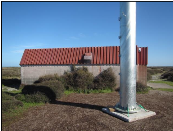
Plate 3: Transmitter building (43 m 2 ) and communications antenna (used by Orion and NZ Police) near the southern boundary of the Concession Area.
