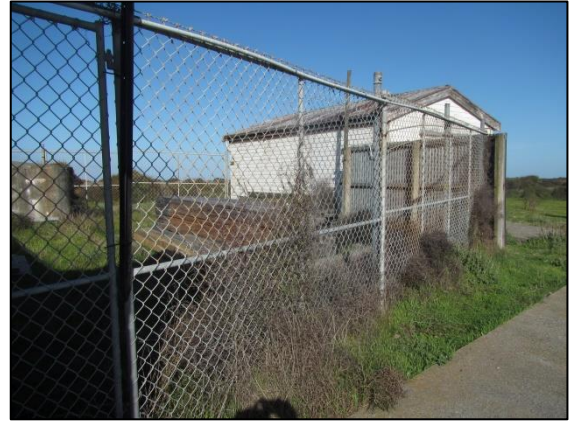
Plate 2: The white shed and fencing are to be removed, as well as stacks of timber and other materials next to the main 'receiver' building.
