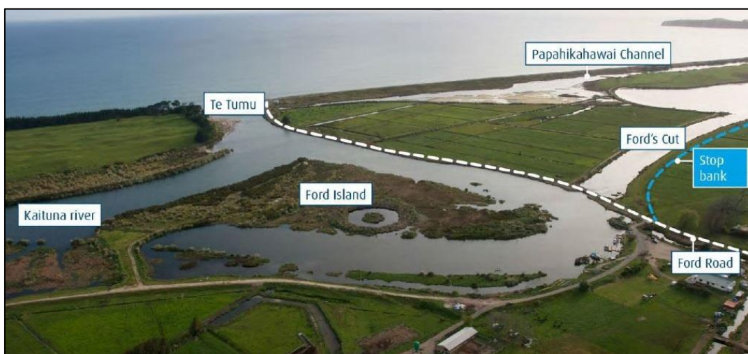
Figure 22: Existing situation at Te Tumu showing the location of channels and stopbanks
