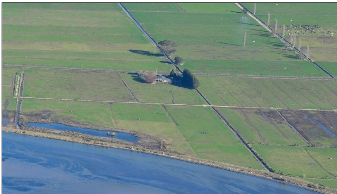
Figure 8: Farm drainage network and stopbanks adjacent to upper estuary
