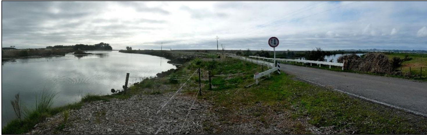
Figure 18: Ford Road at the existing culverts with the Kaituna River
