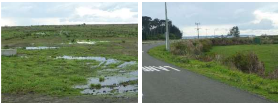
Figure 3 Brain land. In the right hand photo can be seen the green pumpstation discharging under Ford Rd to the river.
