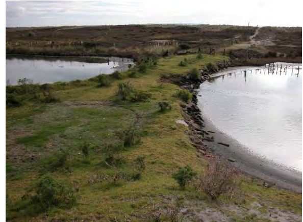
Figure 16 Causeway from Papahikahawai Island to spit impeding tidal flushing of Papahikahawai Lagoon.
