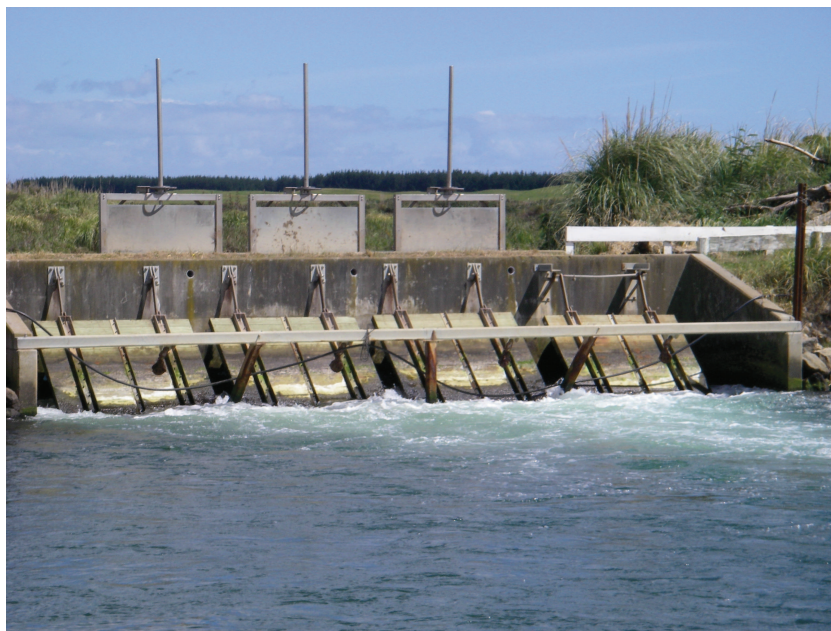
Figure 0-1 Fords Cut Tidal Gates
