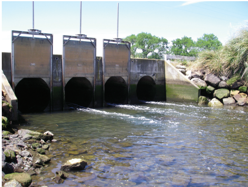
Figure 0-2 Fords Cut Culverts
