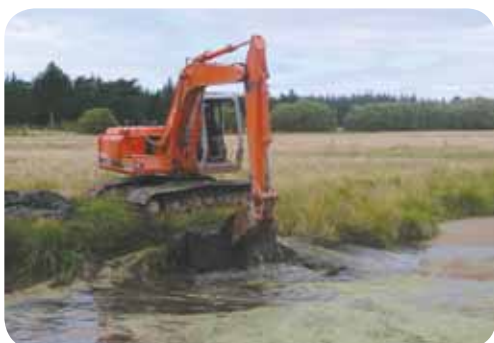
Clearing of a waterway.
