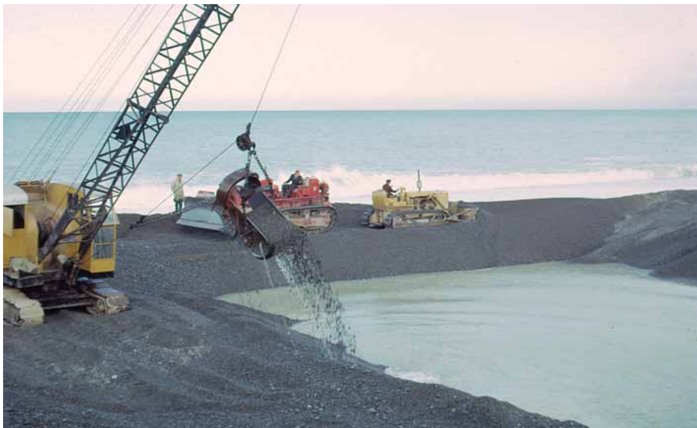
Lake openings, now: Dragline and bulldozers opening the cut at Lake Ellesmere/Te Waihora.
