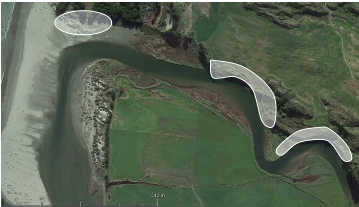
Figure 6: Diagram showing (approximately) the areas assessed as most likely to be affected by river erosion with present river morphology
