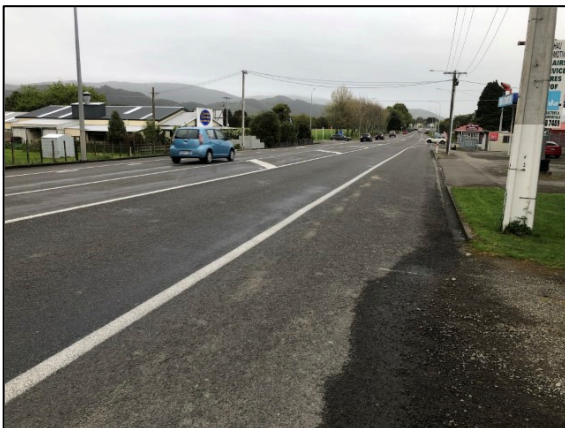
Photo 2.5: View to SW along SH1 towards Muhunua West/East Road intersection
