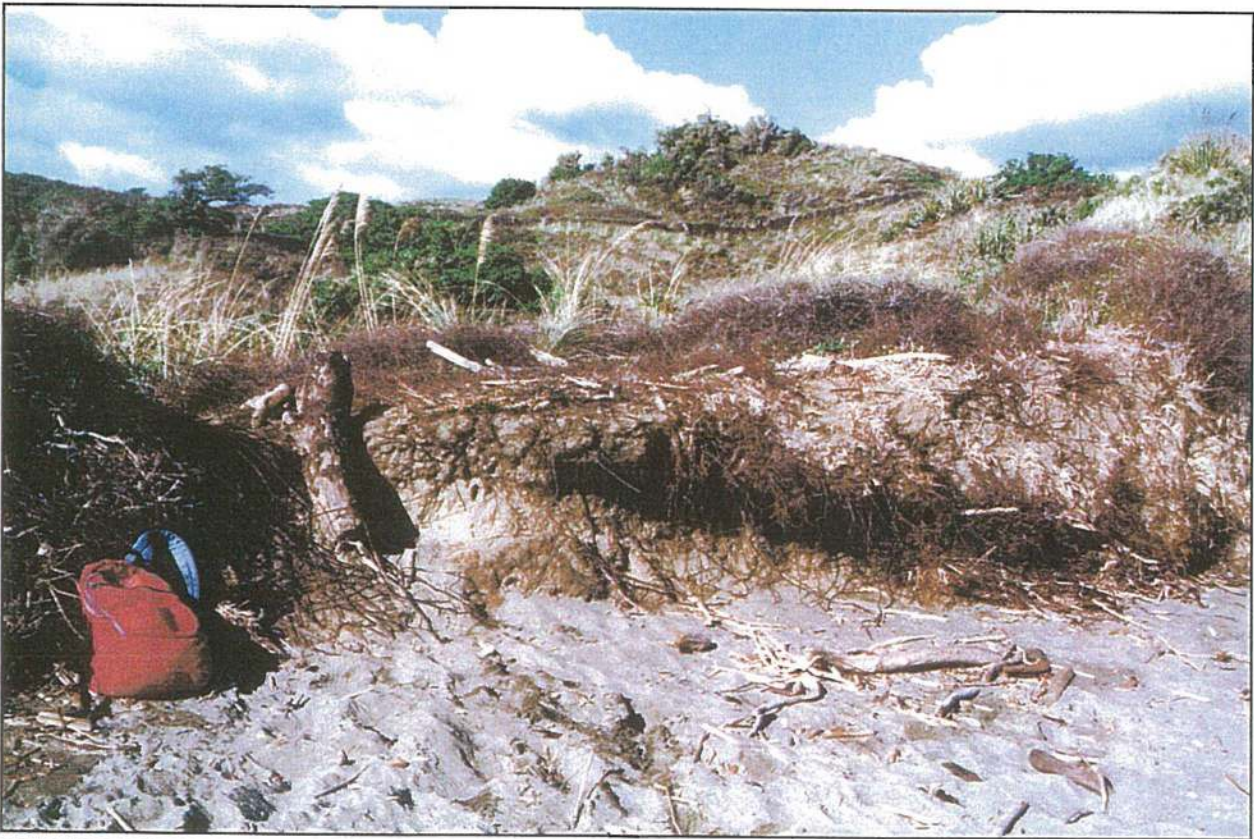
PHOTOGRAPH 10: Simple wooden stepped access could be provided here to avoid erosion at nick-point (behind log) which is present step down point.
