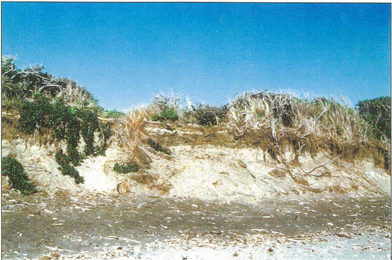
PHOTOGRAPH 4: Eroding inter-dune terrace, between Raumati and Whareroa Stream. Erosion at these points is very difficult to stop and can move the dune edge inland rapidly.
