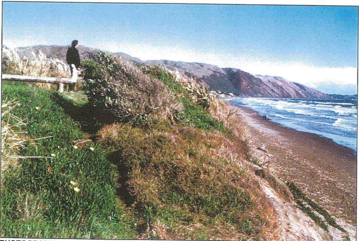
PHOTOGRAPH 6: Semiactive dune edge (right), within a few metres of edge of parking area (left), Wainui area. Even with slower rates of erosion at this end of the park, such areas can be expected to be at risk
