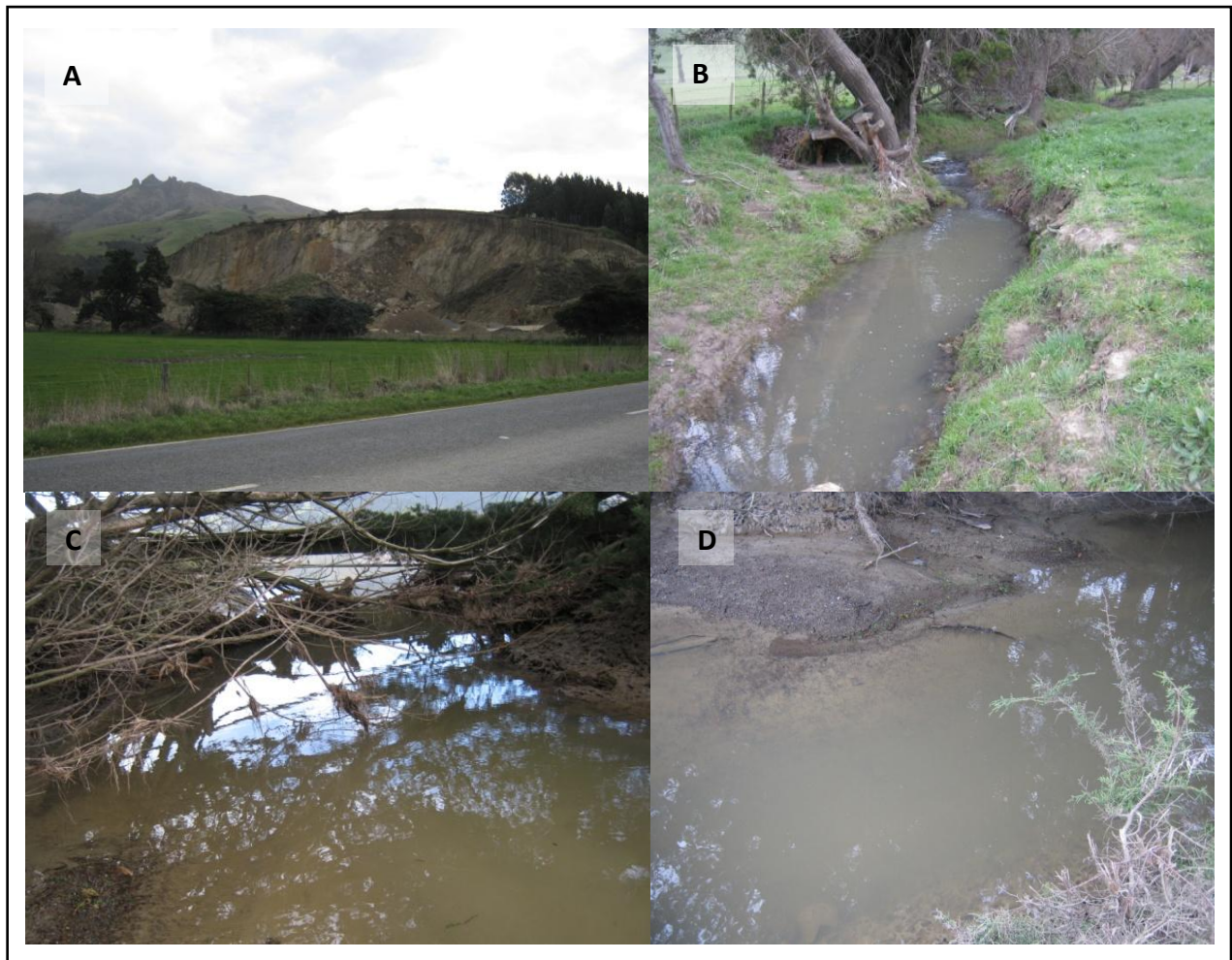
Figure 8. A) The quarry adjacent to Foleys Stream in the Head of the Bay, B) a reach of the stream upstream of the quarry, C) and D) illustrate how the morphology of the channel and flow velocity has changed due to an increase in fine sediments forming a thick layer of mud on the banks and bed. Photos taken 26/8/2010 by M. Shearer.
