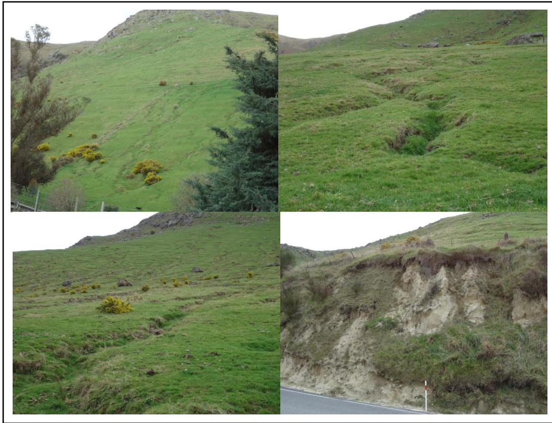
Figure 5. Evidence of soil erosion in paddocks in the Rapaki Catchment and mass wasting from a typical road cutting. Photos taken 10/9/11 by M. Shearer.
