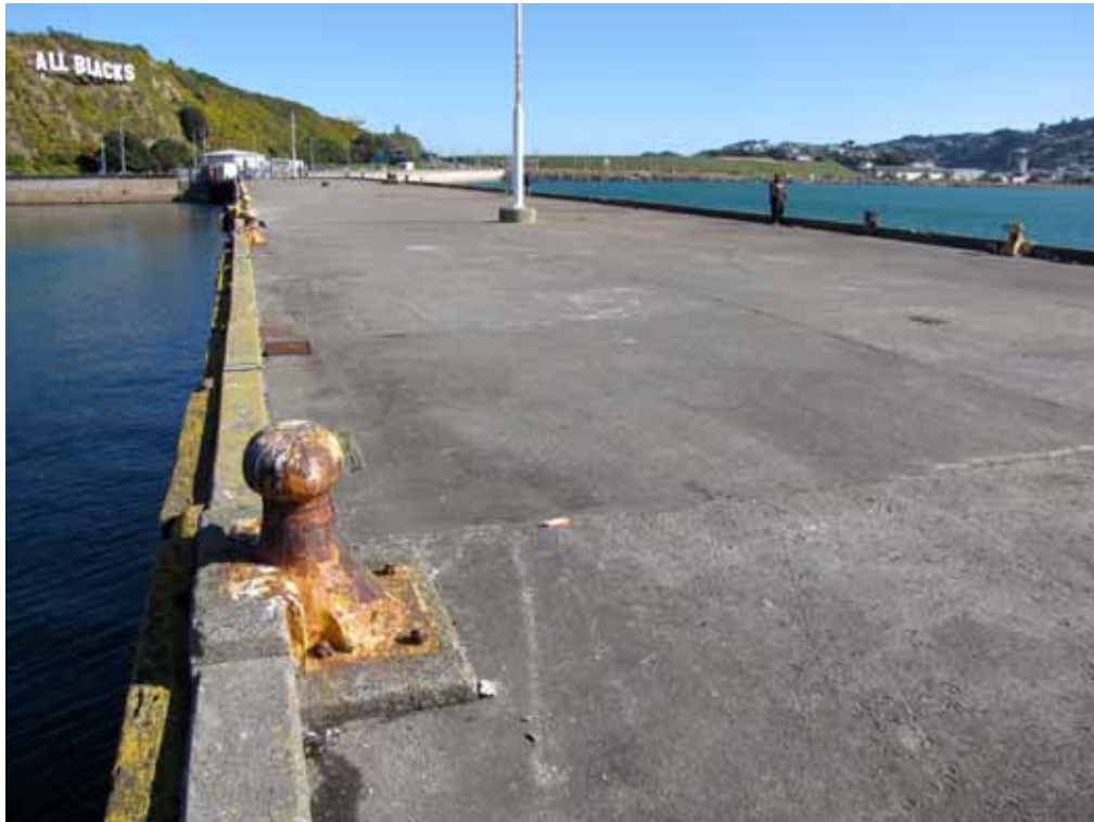
The expanse of the concrete deck of the wharf, looking south
