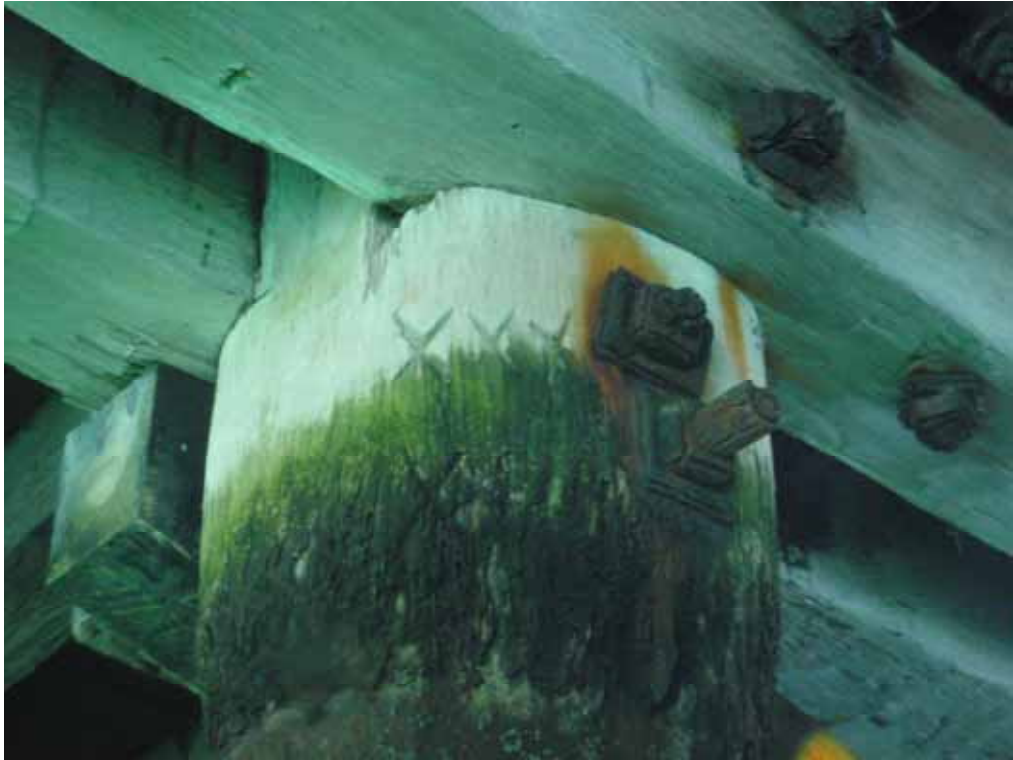
Original timbers bearing assembly numbers in Roman numerals
