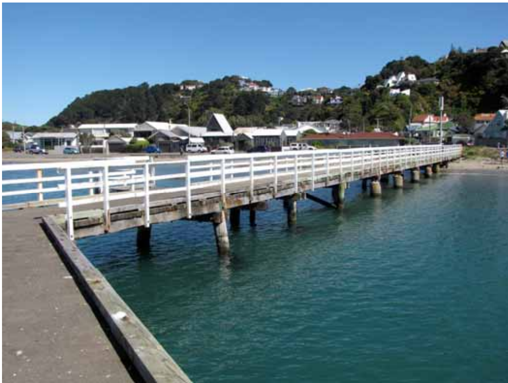
Looking back to the landward end of the wharf
