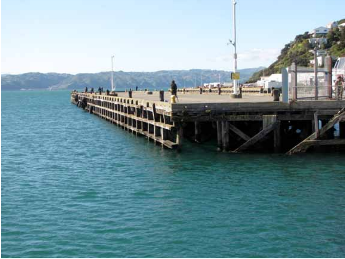
Miramar Wharf, looking north from Cobham Drive, 2012
