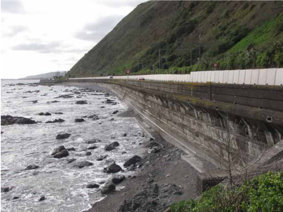
Centennial Highway seawall, near Pukerua Bay
