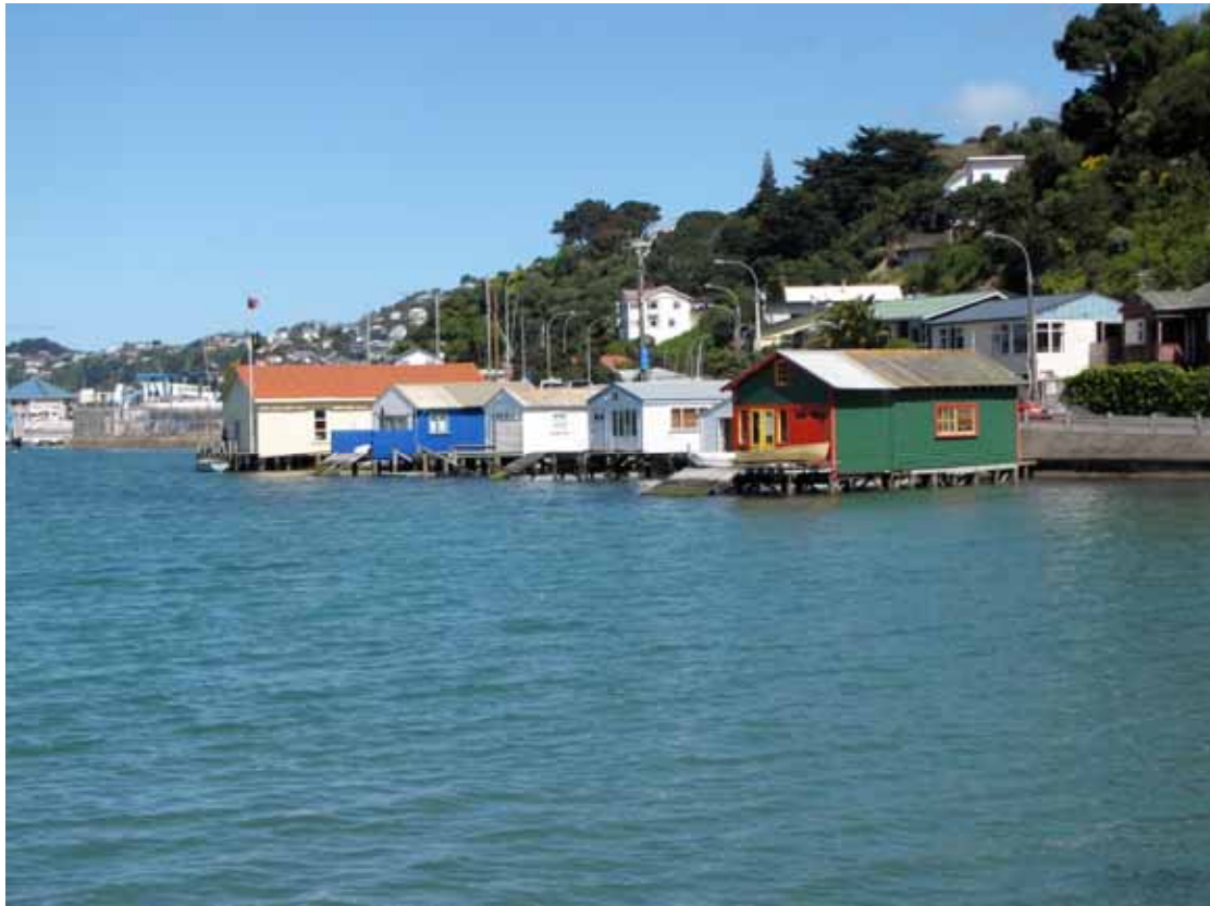
Evans Bay boatsheds, looking across Hataitai Beach from the north
