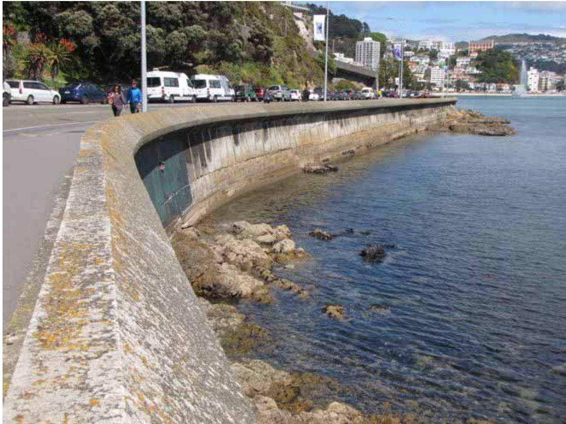
Seawall, near the northern end at Point Jerningham, looking south, 2012
