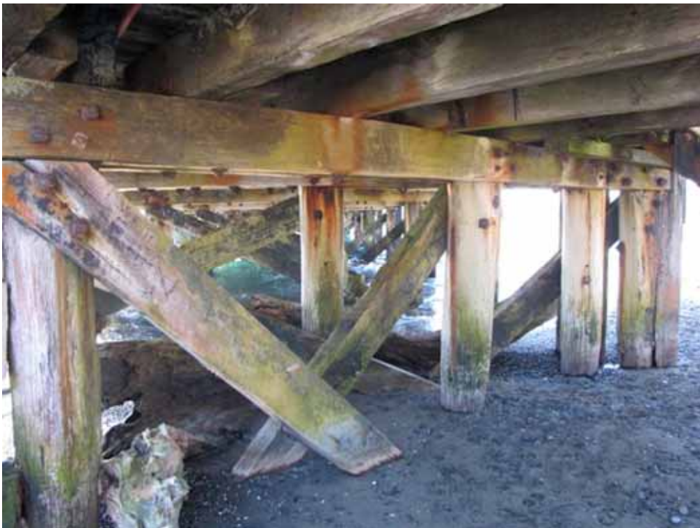
Detail of the piles and below-deck structure of the wharf
