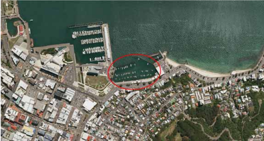
Clyde Quay Boat Harbour – former Overseas Passenger Terminal (and Clyde Quay Wharf) to the left of the harbour, Freyberg Pool to the right. Image from Google Maps, 2012
