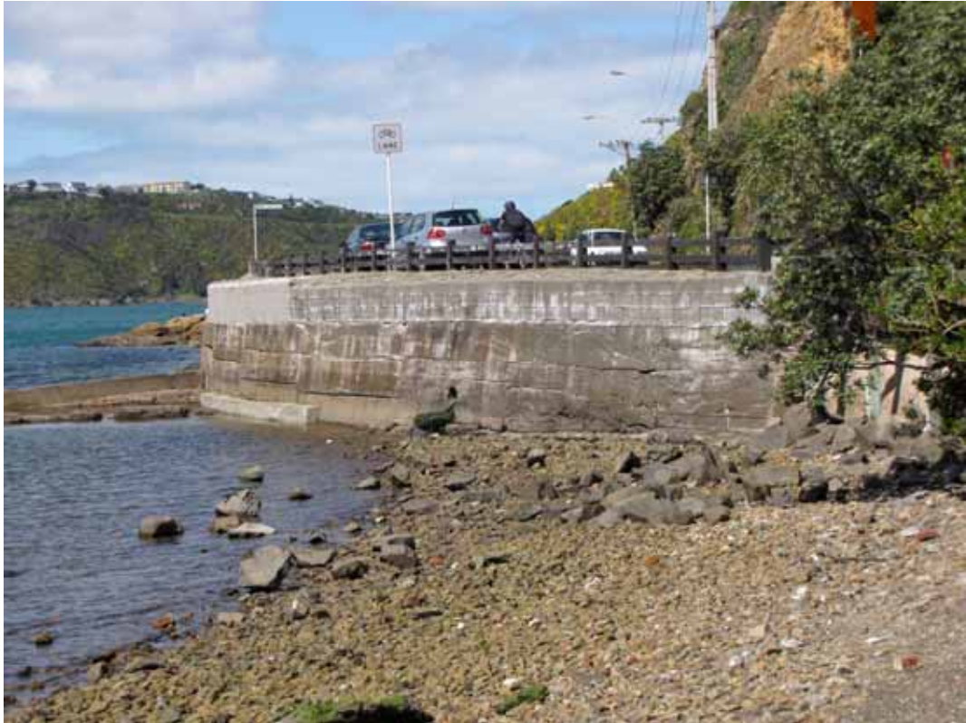
Seawall at the south end of Balaena Bay.
