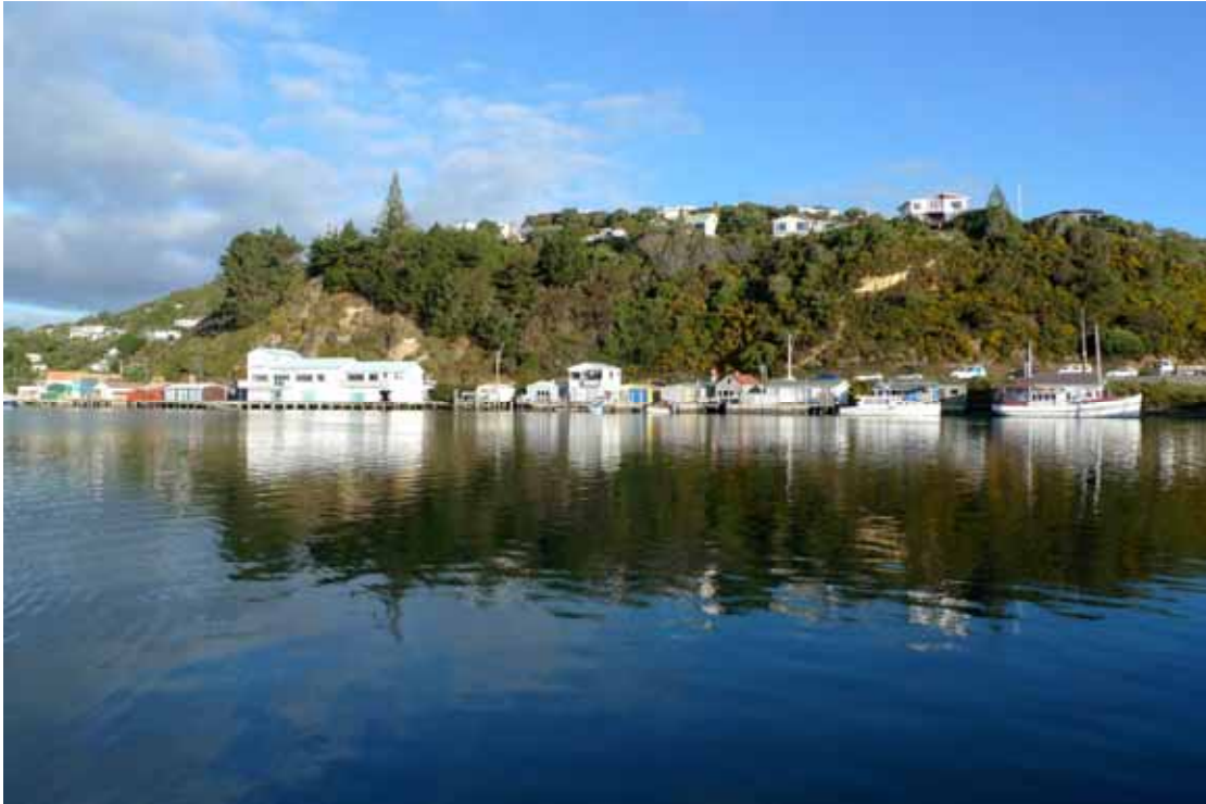
Boat Sheds, from the Paremata Road Bridge, 2011
