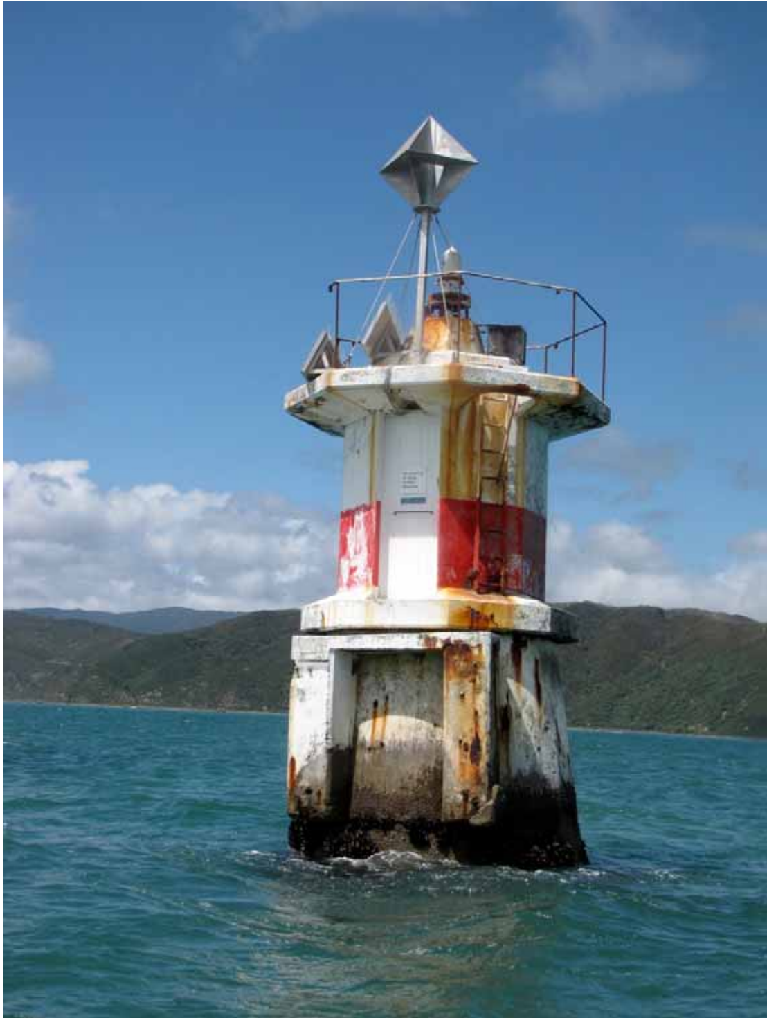
The north-western side of the light with the Eastbourne hills beyond
