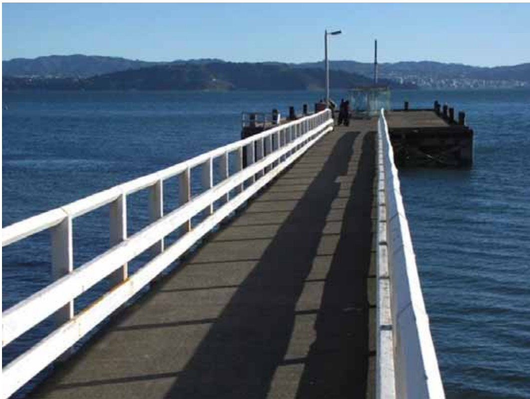
Days Bay Wharf, from landward side looking out to sea, July 2011
