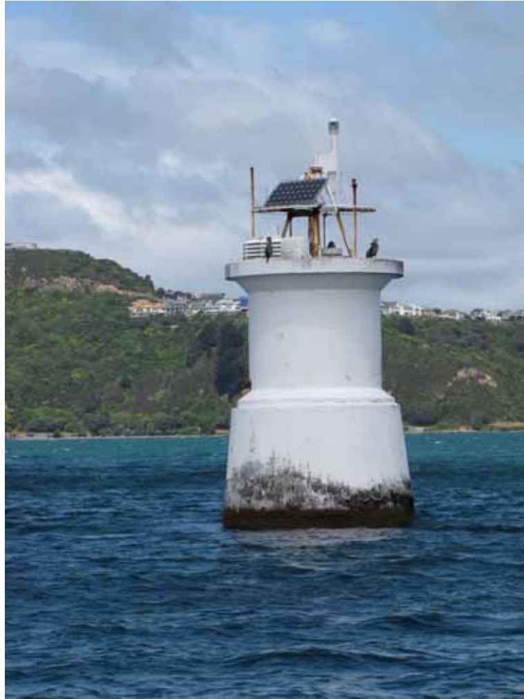
Point Jerningham Light, Miramar Peninsula behind, November 2011
