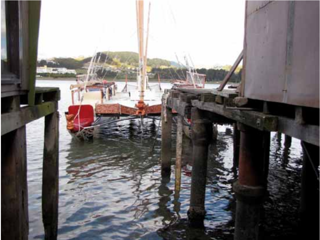
View between two sheds; note the pile formers made of earthenware pipes
