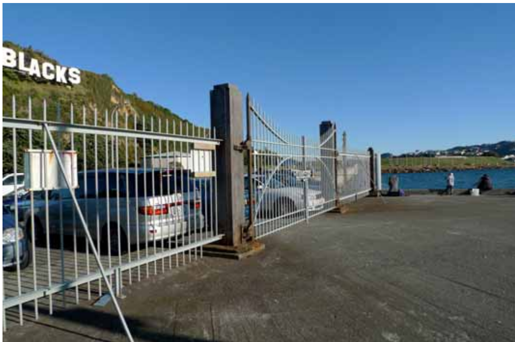
Modern wharf gates hung on the original gate posts and gate stiles
