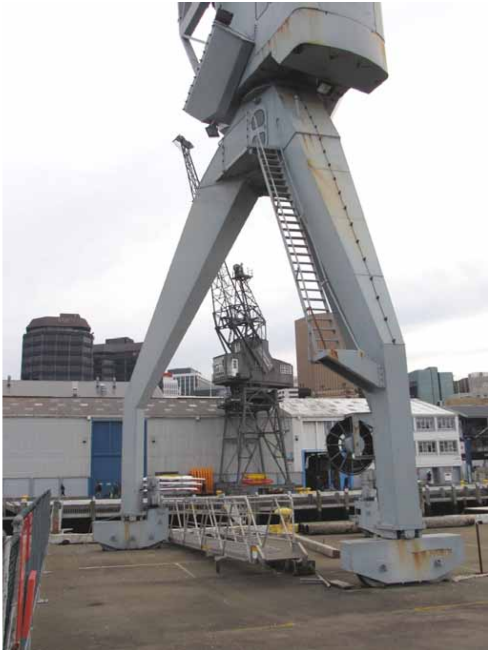
The level-luffing crane, 1951, seen through the legs of the tripod crane, 1966
