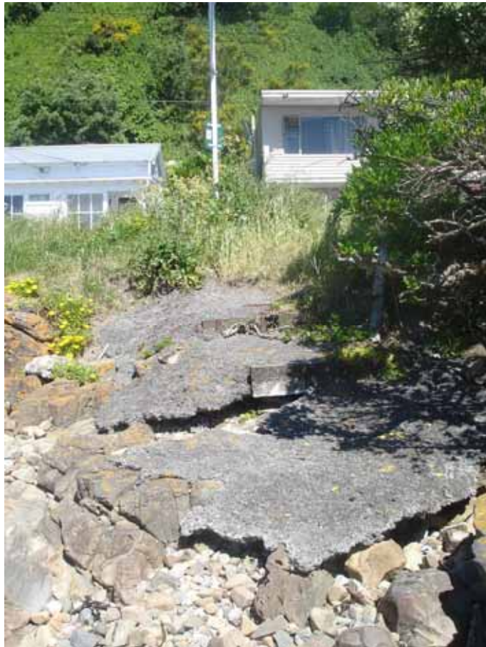
Ancillary concrete work, just up the bank from the obstacles
