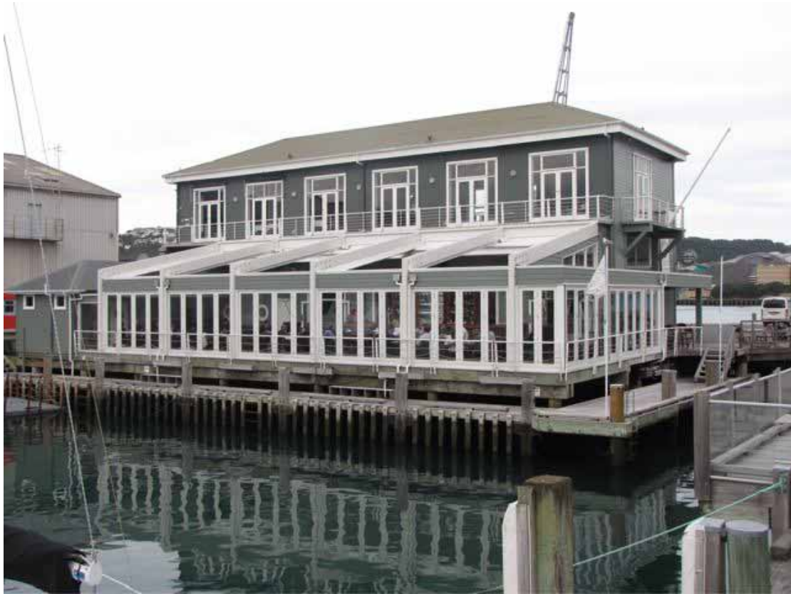
Shed 3, from the west, 2012
