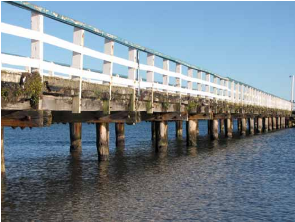
Close-up view of the west side of the wharf structure
