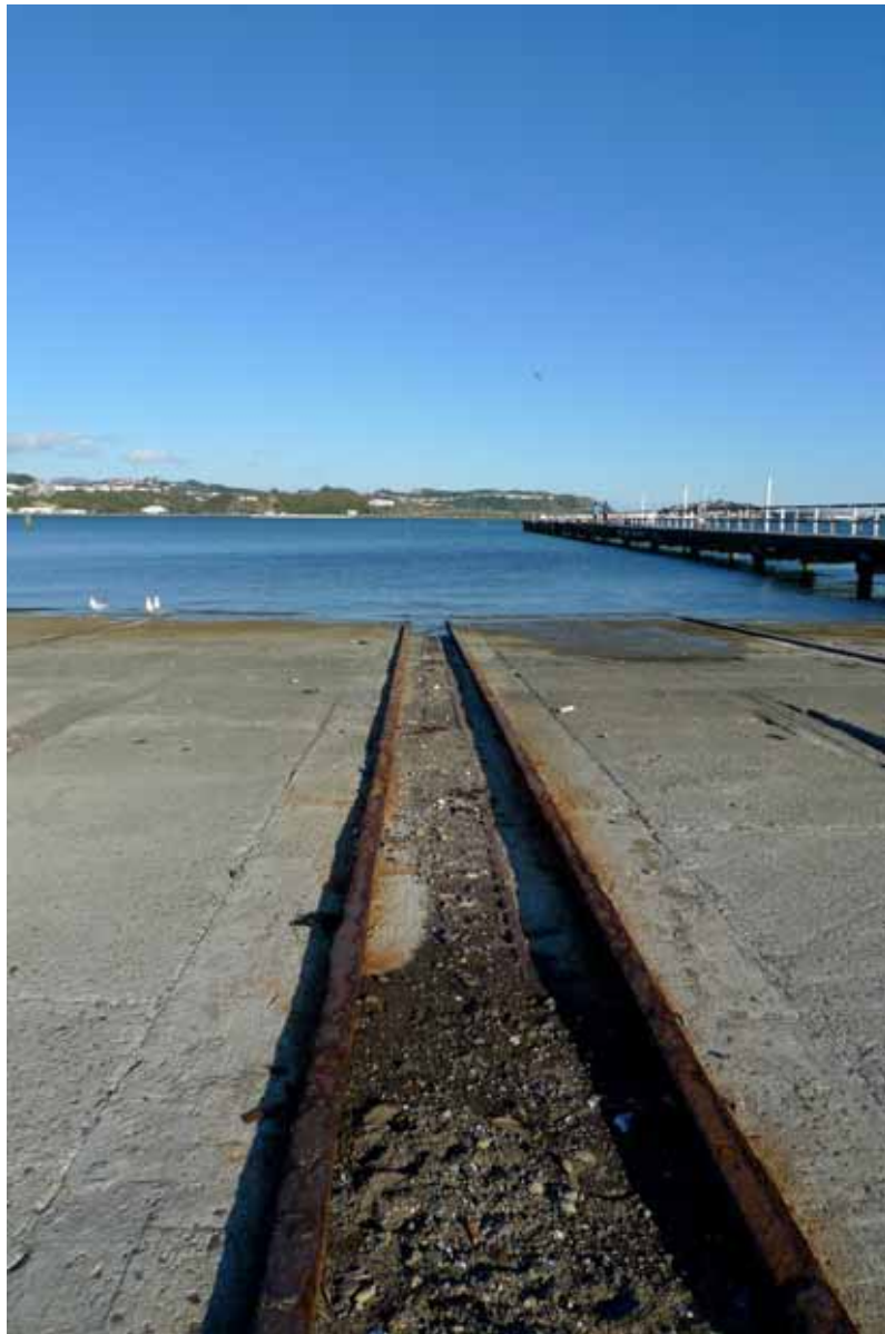
No. 2 slipway and wharf, 2012
