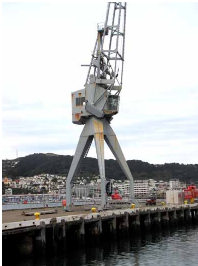
Outer tee, eastern section, showing helipad area and tripod crane, 2012
