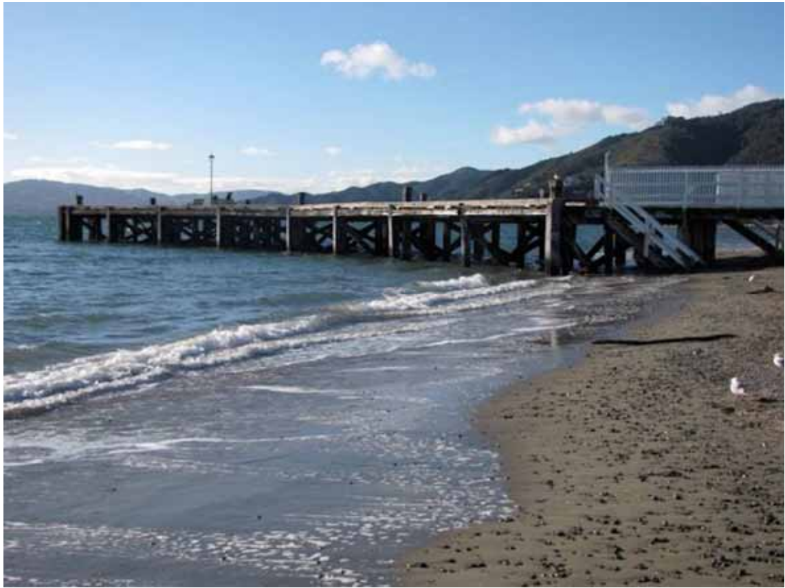
Rona Bay Wharf, from the south, July 2011
