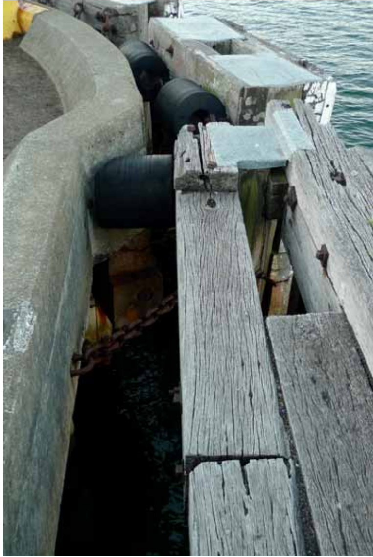
Detail of heavy timber buffers, near north end
