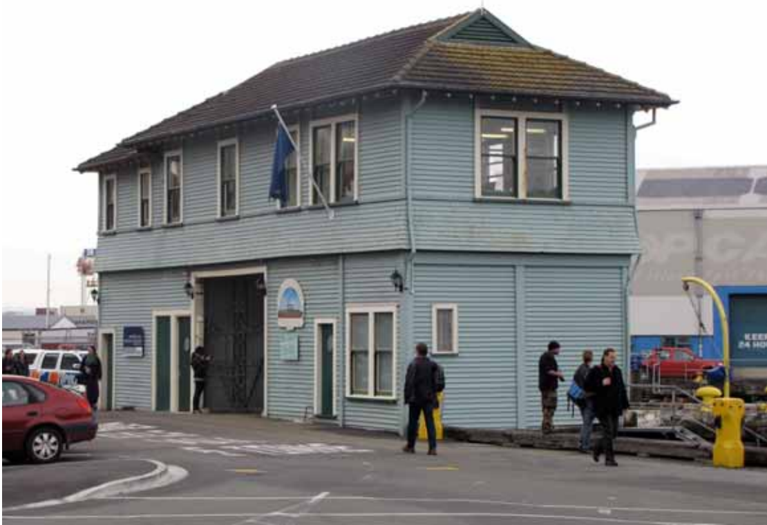
Eastbourne Ferry Terminal, from south, June 2011
