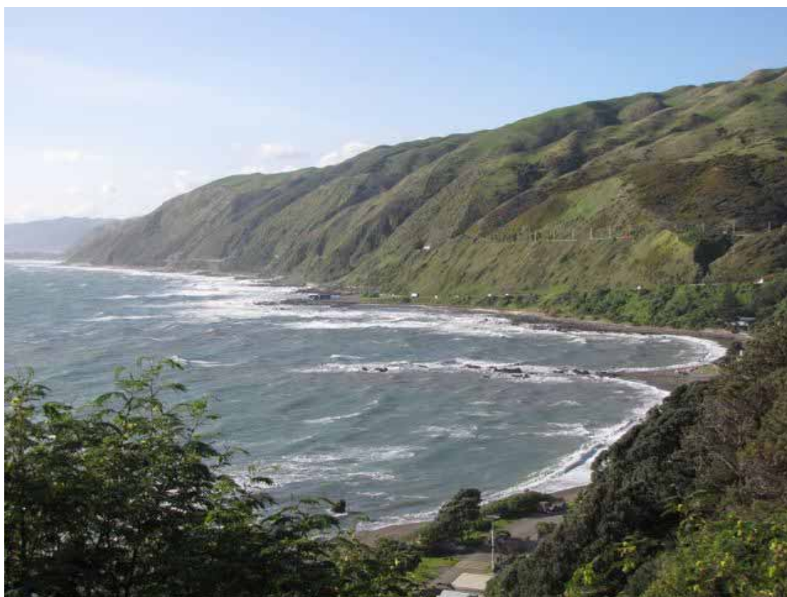
The rugged coastal setting of the Centennial Highway from Pukerua Bay. The sea wall starts to the north of the point in the middle of the image.
