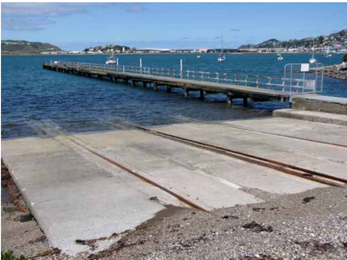
No. 2 slipway as it enters the water
