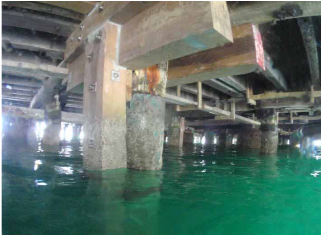
Modern repairs alongside original timber elements
