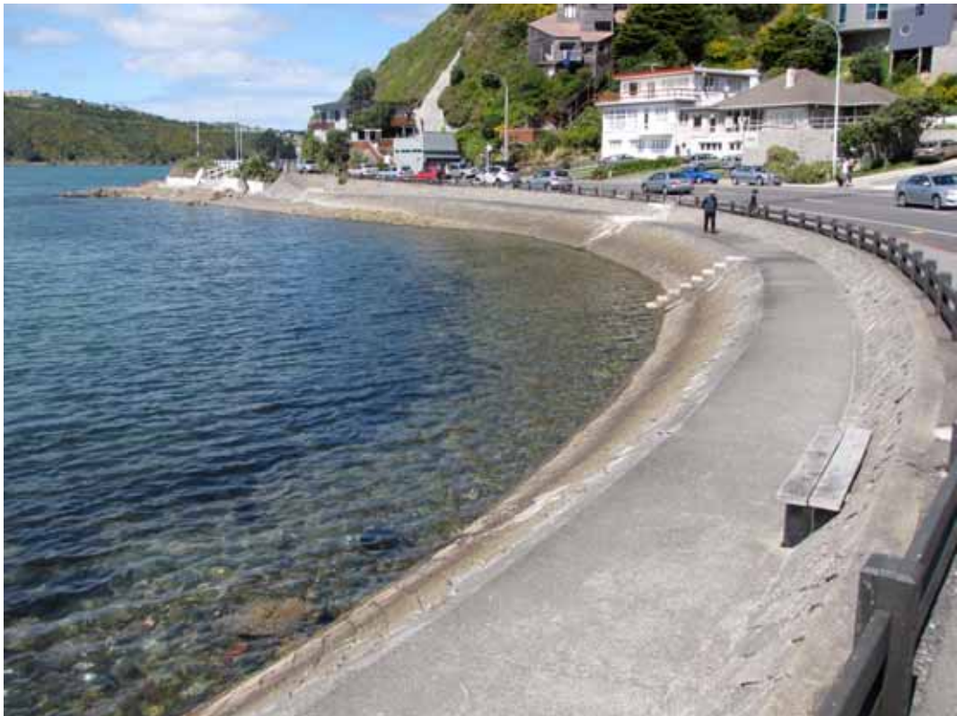
Seawall at Weka Bay.
