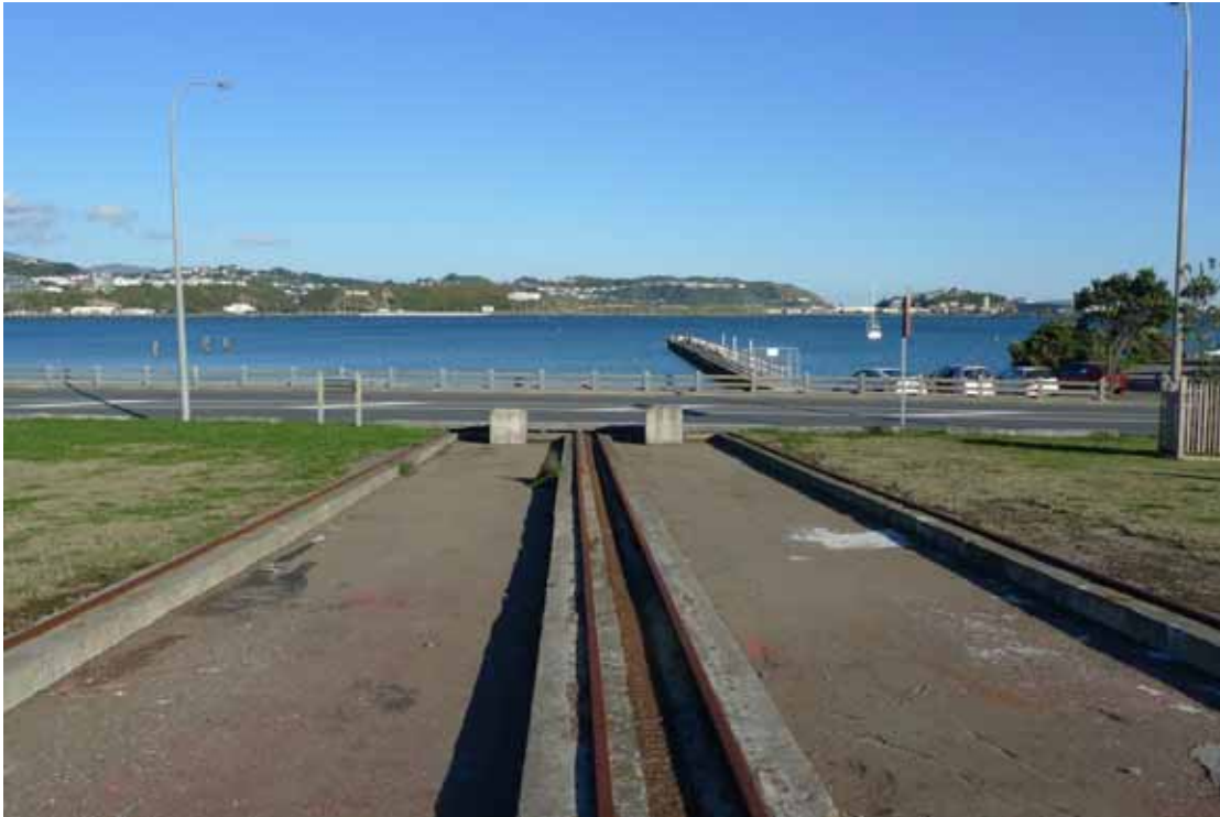
Upper part of No. 2 slipway, wharf in the distance. Note how the elevated road cuts off the visual continuation of the slipway to the sea
