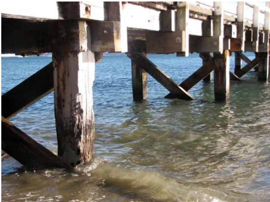
Detail of the structure of the Days Bay wharf, July 2011
