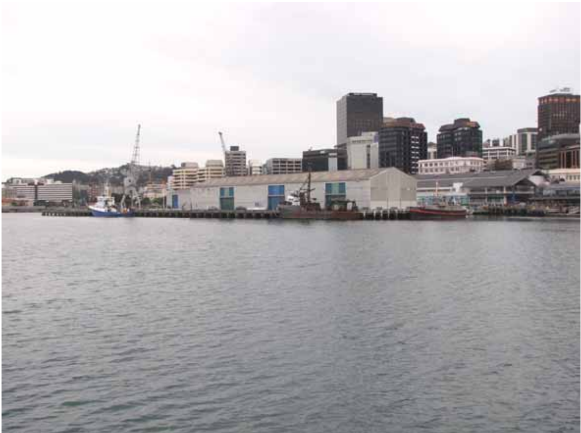
Queens Wharf, from the north, 2012
