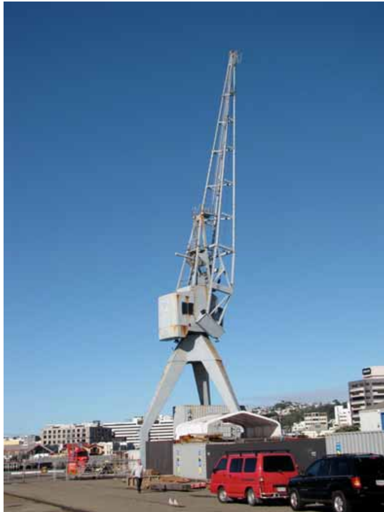
The tripod crane, 1966, on the outer Tee of Queen's Wharf.
