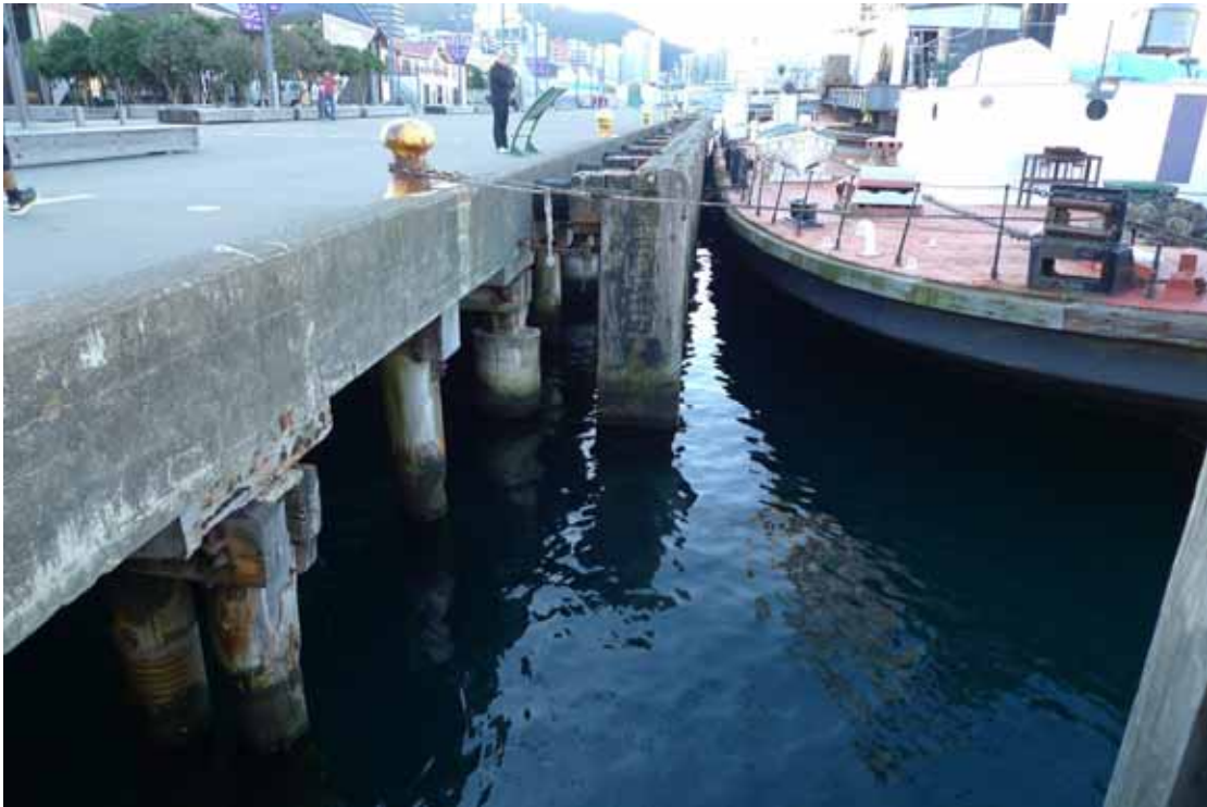
Sub-structure, south end – note concrete casing around alternating piles
