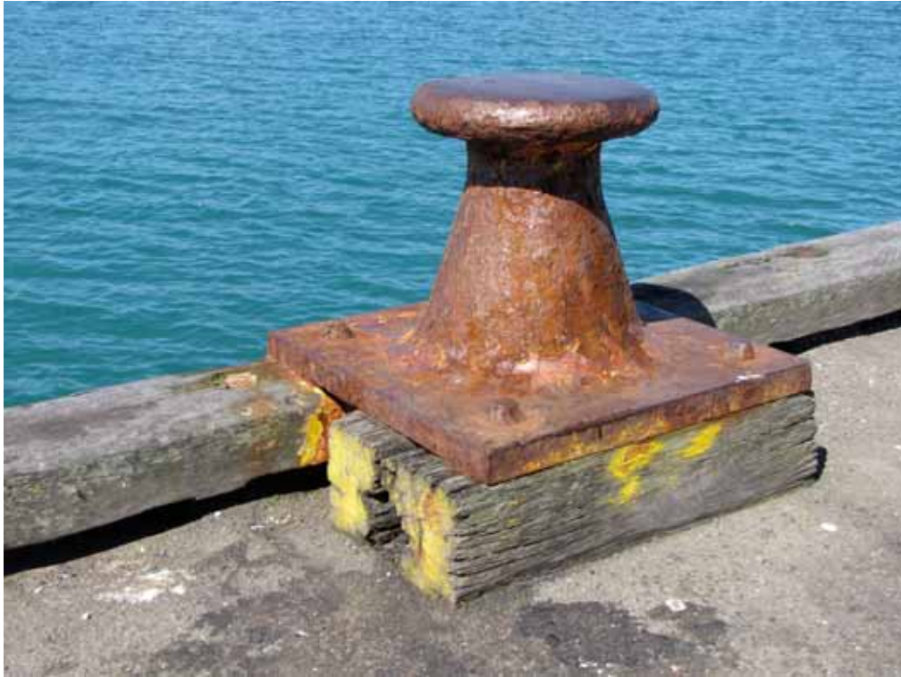
Cast iron bollard, eastern side of wharf
