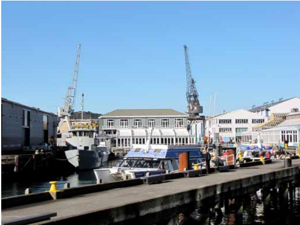
Shed 5 in context from the north, March 2012, showing the two cranes and Shed 1 (left), Shed 3 (centre) Shed 6 (to the right of Shed 3) and the Queens Wharf events centre looming in the background
