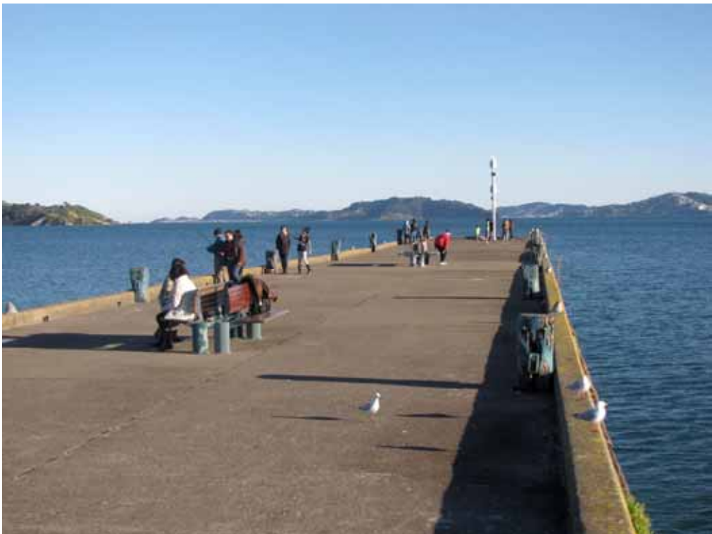
The wider outer end of the wharf, now decked in concrete
