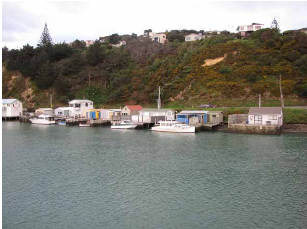
Western end of the group of boat sheds, June 2011
