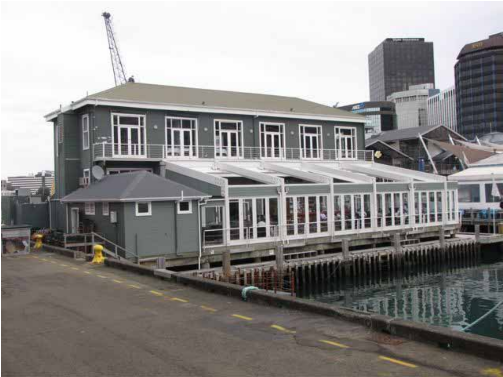
South elevation, June 2011
