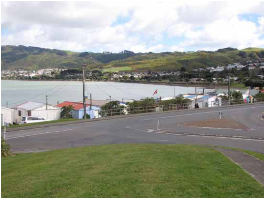
Roofs of the boatsheds from the landward side
