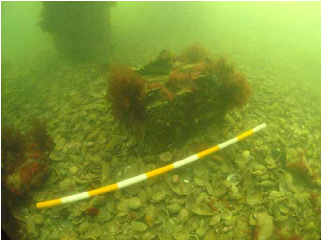
Truncated wharf pile with copper sheathing beneath the wharf, August 2012
