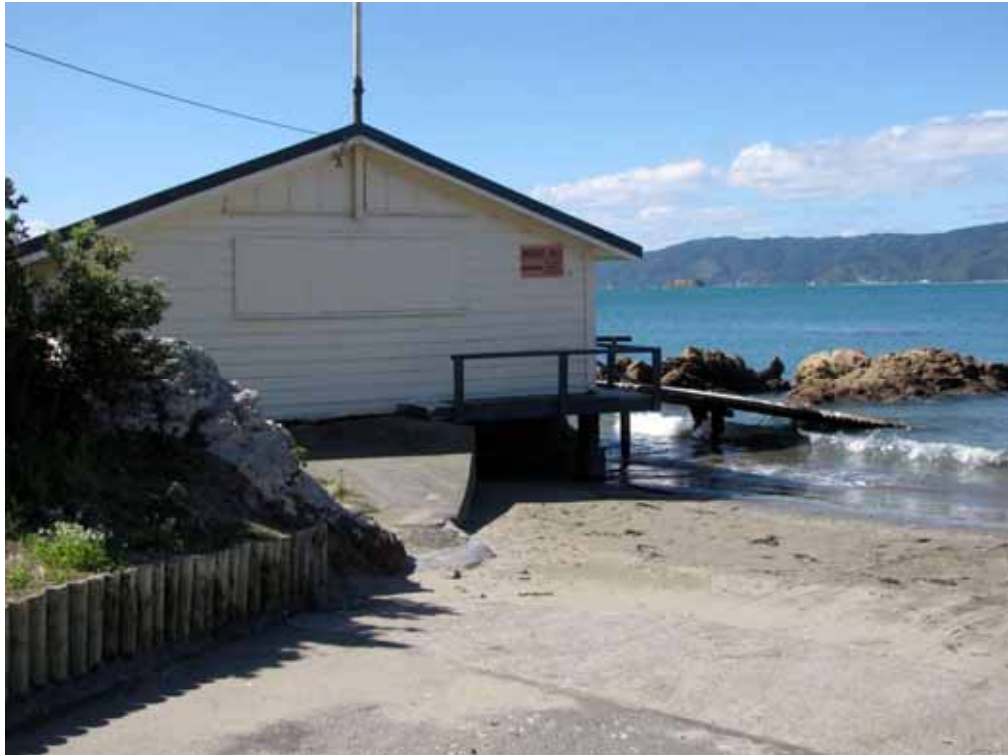
The landward (or south) elevation of the boathouse; concrete launching ramp in the foreground.
