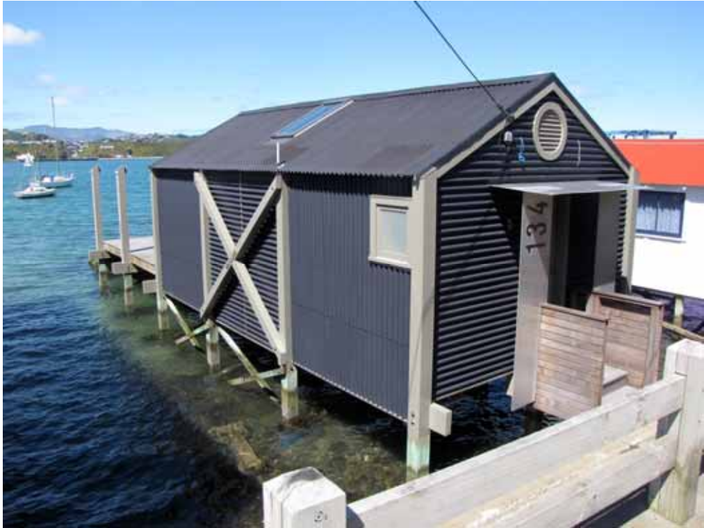
A modern shed, no 134.
