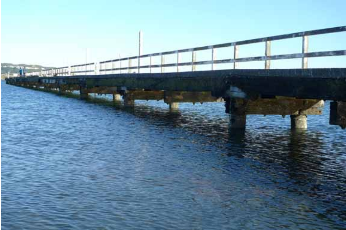
The wharf and its substructure
