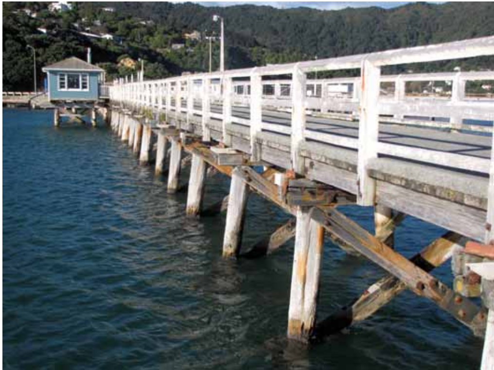
Northern edge of the main part of the wharf.
