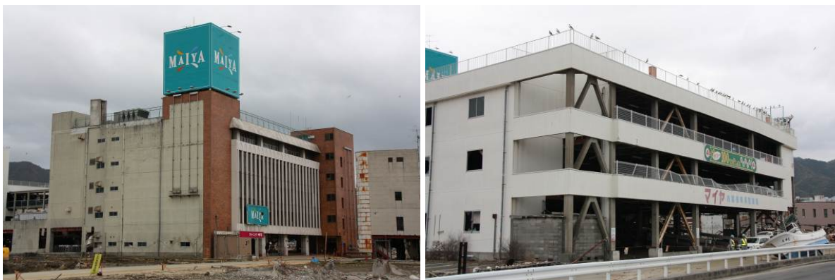
Figure 39 Maiya shopping centre, which was inundated to the 3 rd storey
