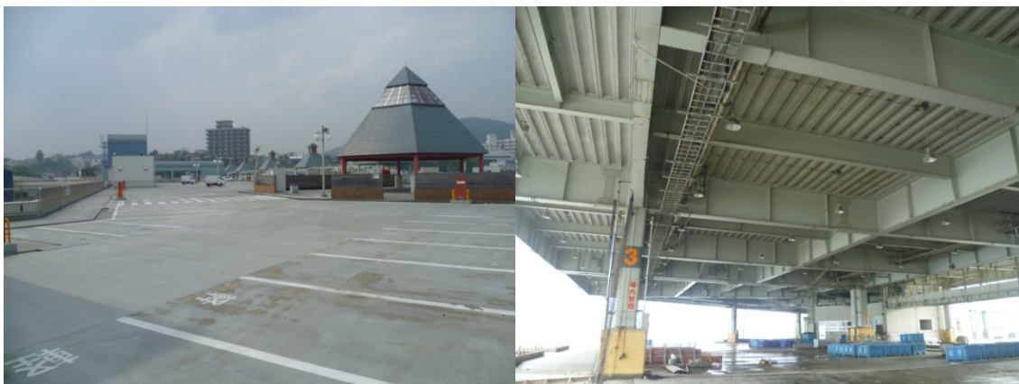
Figure 49 The large open car park roof space above the fish market provided refuge to 1000 people. This structure is at the harbour front and inundation almost reached roof level. The open steel structure enabled tsunami flow at the 1 st storey.
