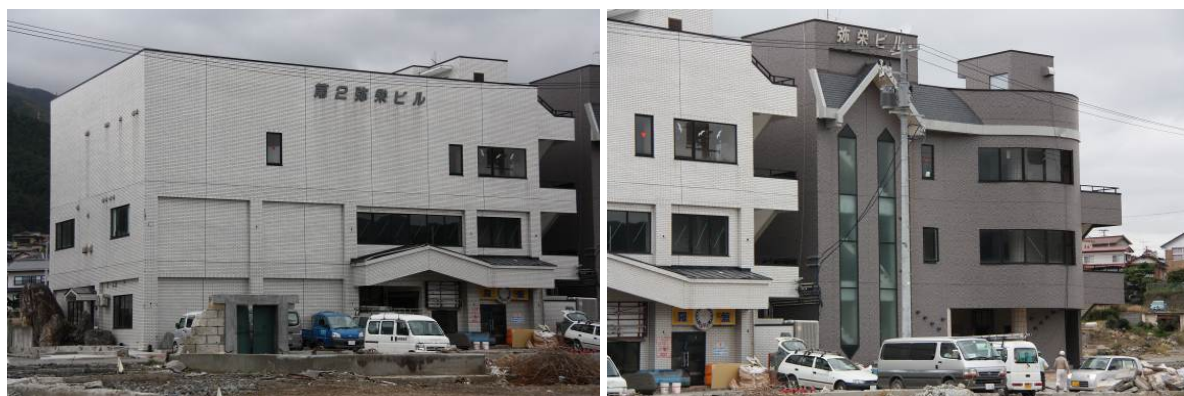
Figure 41 Yasuka private commercial and apartment block number 1 shows very little exterior damage.
