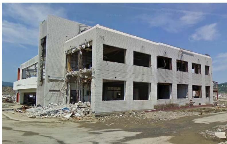
Figure 59 Minami-Sanriku fisheries co-operative building which was overtopped on March 11 th . Image credit: Google Streetview, August 2011.
