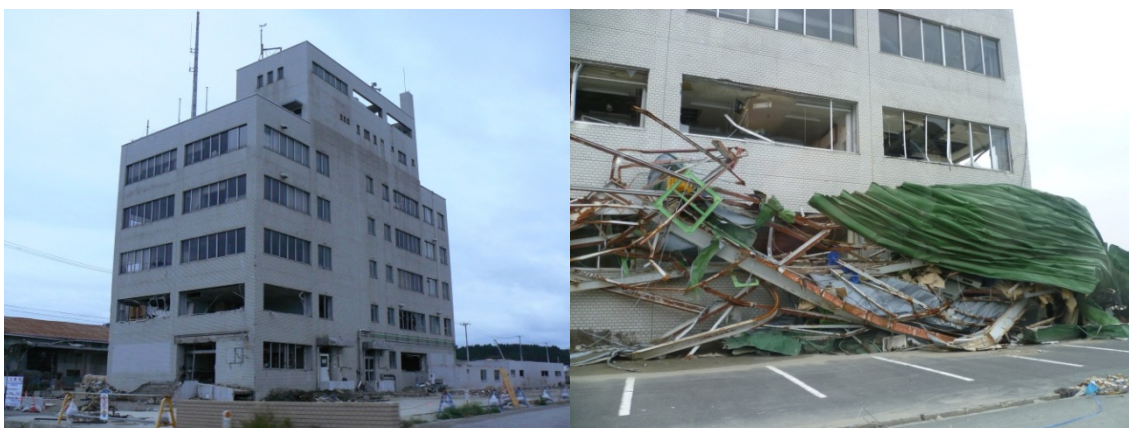
Figure 51 The National Government office, where 120 people took refuge from the tsunami. This building is adjacent to the Prefectural Government offices and was left undamaged when light steel structures were washed into it. The lower two storeys were inundated.
