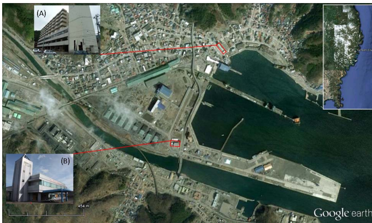
Figure 34 Designated evacuation locations in Kamaishi City. An estimated 50 people evacuated to this apartment block (A) and government offices (B). The entire area shown was inundated; inundation depth was 8 m in the vicinity of building (A).
