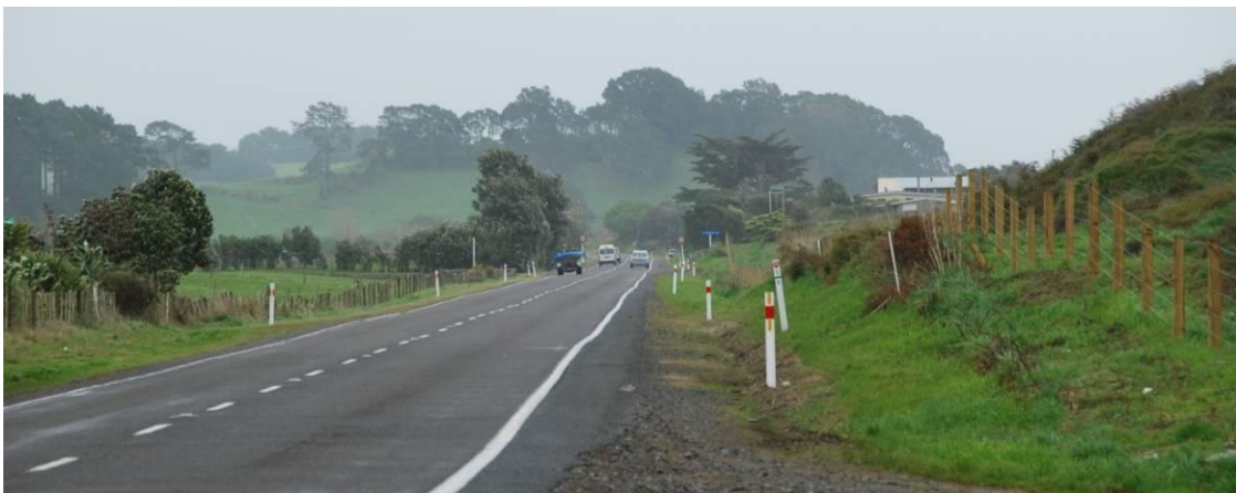
Figure 4: State Highway 35, looking west to Tablelands.
