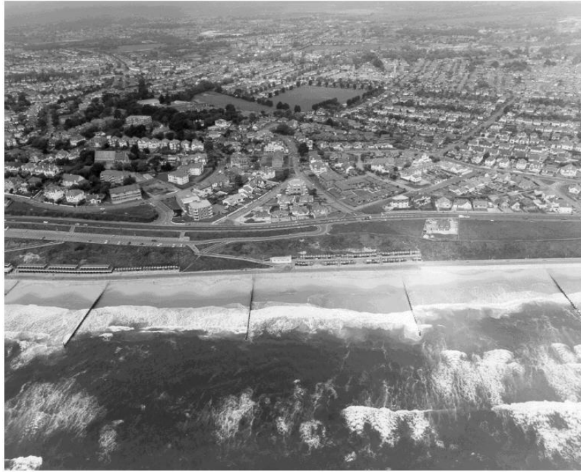
Figure 7. An aerial view of the successive groynes in Poole Bay.
