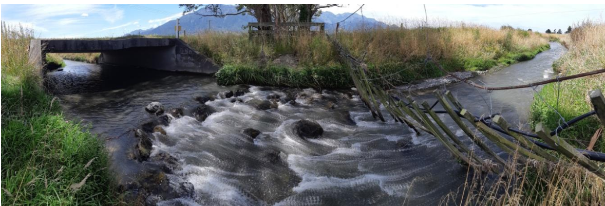
Fig. 4. A remediated section of Middle Creek where a bottom slope was installed at a small pour-over downstream of the State Highway 1 bridge. Photo: Heath Melville.
