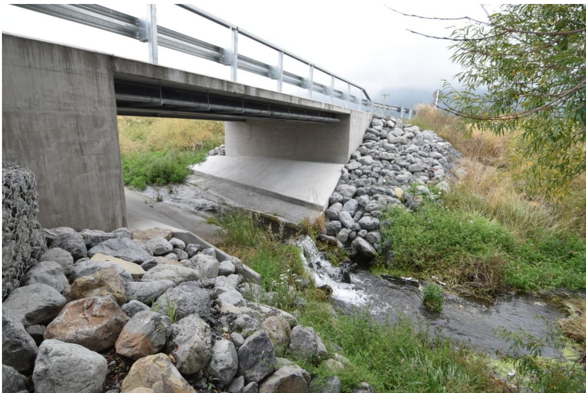
Fig. 2. A suspected fish passage barrier at Mt Fyffe Road bridge associated with a vertical headwall.
