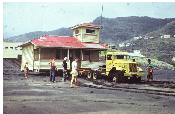
Figure 3.5 - Removal of the original club with the new club in distance
