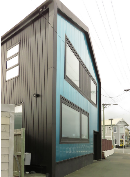
figure 6.8 Lyall Bay renovation
