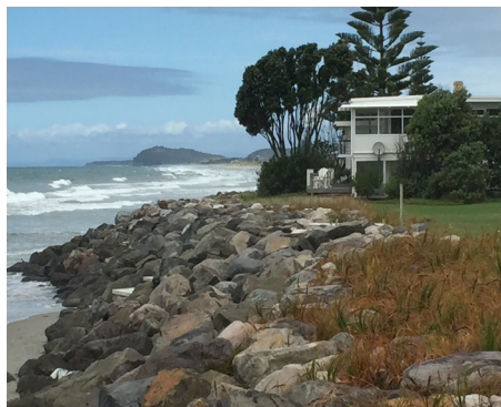
Figure 3: Waihi Beach rock buttresses
