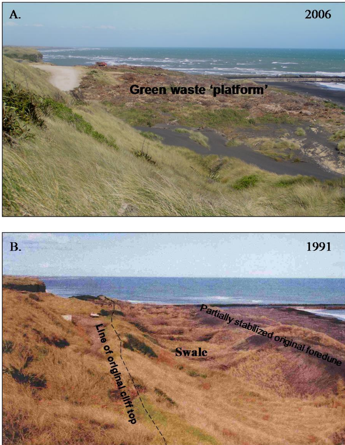
Figure 12 By 2006, a green waste 'platform' had been created (A) by infilling the swale between the original cliff and the crest of the original foredune (B). Note drift-sand at northern margin (in foreground) of green waste platform in A.
