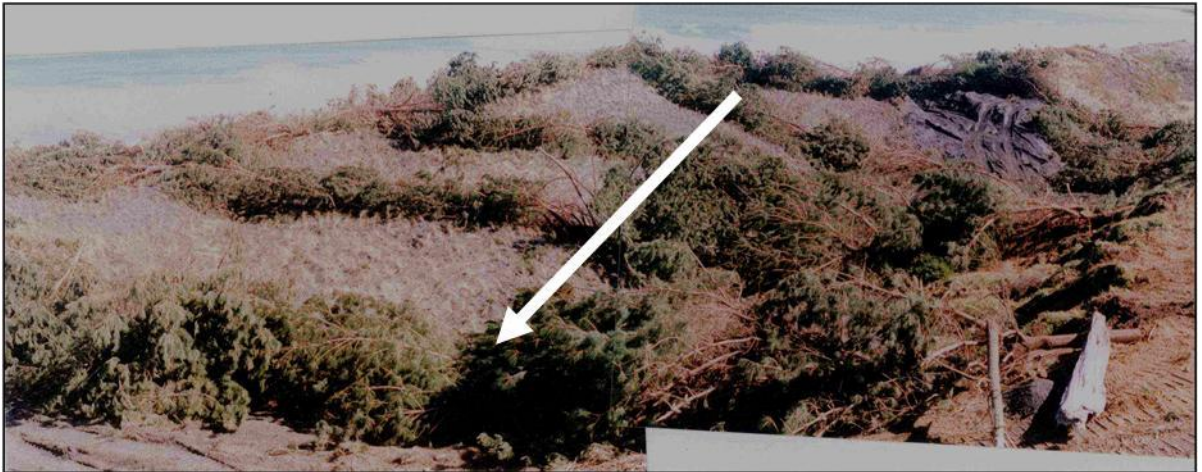
Fig 10 Sand stabilization works carried out in 1988. Pine thinnings were placed in gullies and across the path of the prevailing wind (see arrow), with marram planted within the intervening spaces.
