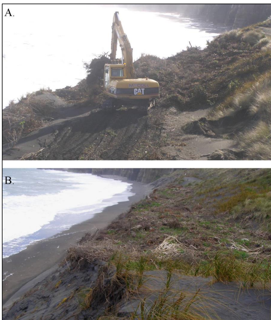
Figure 13 Green waste being placed along the scarp-top (A) in July, 2014. NB the extent of this scarp is evident in Figure 5. The stabilizing effect of the green waste treatment compared with vegetation (pingao) cover is indicated in B (October, 2014) where the pingau area in the foreground has greater scarp retreat and associated landward wind-drift.
