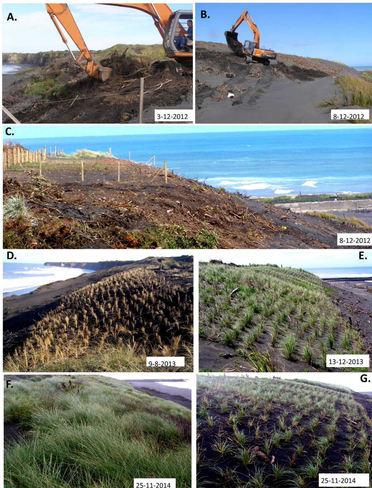
Figure 17 Marram block planting. Site preparation (A to C) carried out in December 2012 (fence and surface contouring). The 2013 planting is shown in D, after 4 months growth in E, and after 15 months in F. The 2014 planting after 4 months is shown in G with the 2013 planting visible in the distance. Locations are shown in Appendix B7 and B8.
