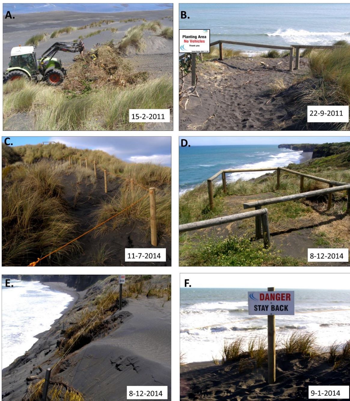
Figure 30 Access control using green waste barrier (A), post and pole barrier and sign at Upper Carpark entry to Upper Basin (B), and perimeter pedestrian fence around Upper Basin (C). Expanded barrier fence and upper car park entrance to allow for view (D). The hazard fencing along top of erosion scarp (E) and hazard sign at top of erosion scarp (F) has had to be relocated on several occasions as erosion progresses landward.
