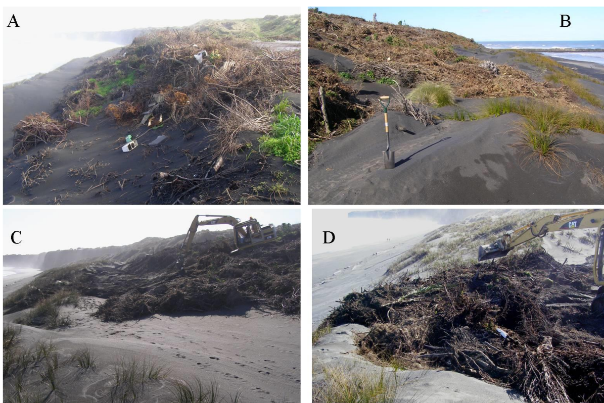
Figure 12 Green waste placement. Recently pushed to the front of the platform face in the Central Sector (A) with an earlier placement and sand infill in foreground. Green waste spilling down face of platform and across swale (B), and subsequent swale clearance (C) with waste being placed in guts on top of the pingao foredune (D)
