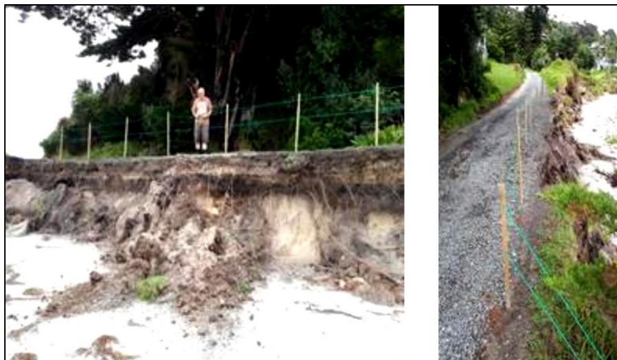
Figure 2 Post-storm erosion threatening DOC access road between Rangiputa settlement and Puwheke Beach, Northland Photos supplied by DOC staff
