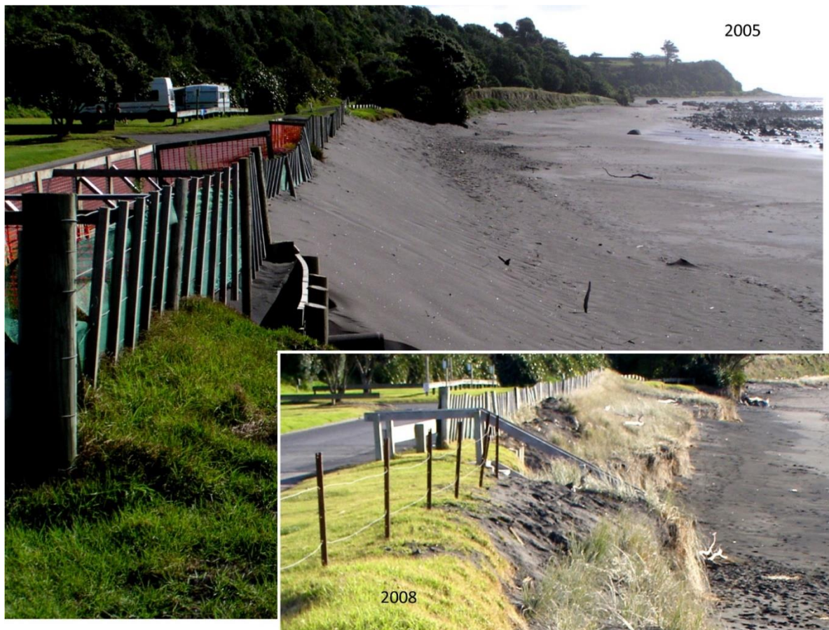
Figure 15 Sand nourishment (push-up) filling the scarped back-shore at Oakura Beach, Taranaki, 2005. A sediment deficit was causing an erosive fluctuation and threatening the motor camp access road. Dune grass was subsequently planted on the push-up to trap wind-blown sand. This management action prevented a significant erosive episode in 2008 reaching the 2005 scarp line (inset). Photos CSL 2005
