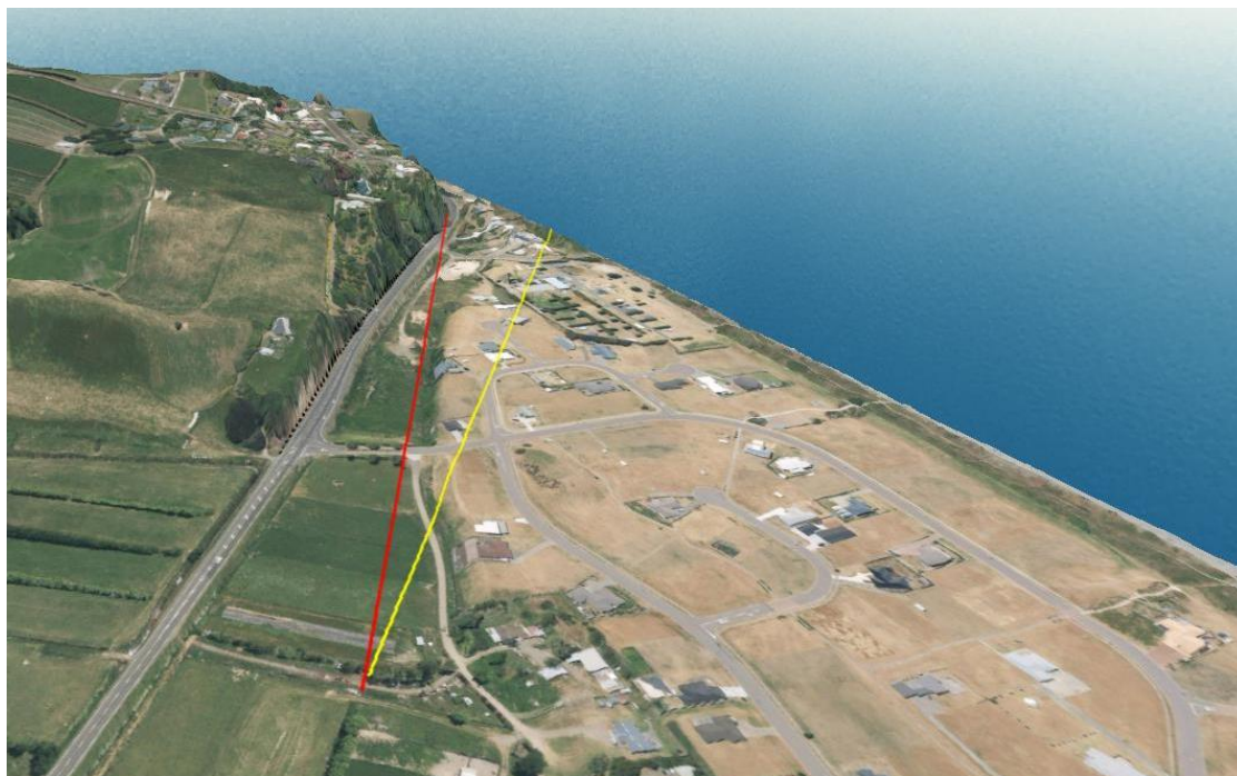
Figure 3 State Highway 2 approaching Waiotahi Beach with old sea-cliff on the left (inland) side of the road. The Waioeku Rivermouth is to lower right off photo (1 km distant). The red line is parallel to the present channel approach alignment (red line in Figure 2), while the yellow line is parallel to the 1985 approach channel alignment in Figure 2. See text for discussion.
