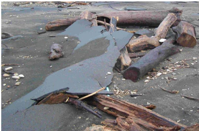
**Figure 22** Delamination of road paving by dynamic inundation flow.
