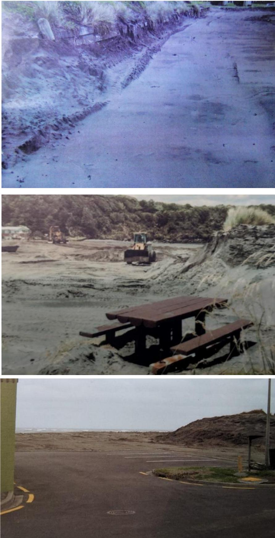
**Figure 11** Mechanical sand removal. Top photo: beach scraping 1990s; middle photo: dune removal 1987, and bottom photo: dune removal 1996-1997
