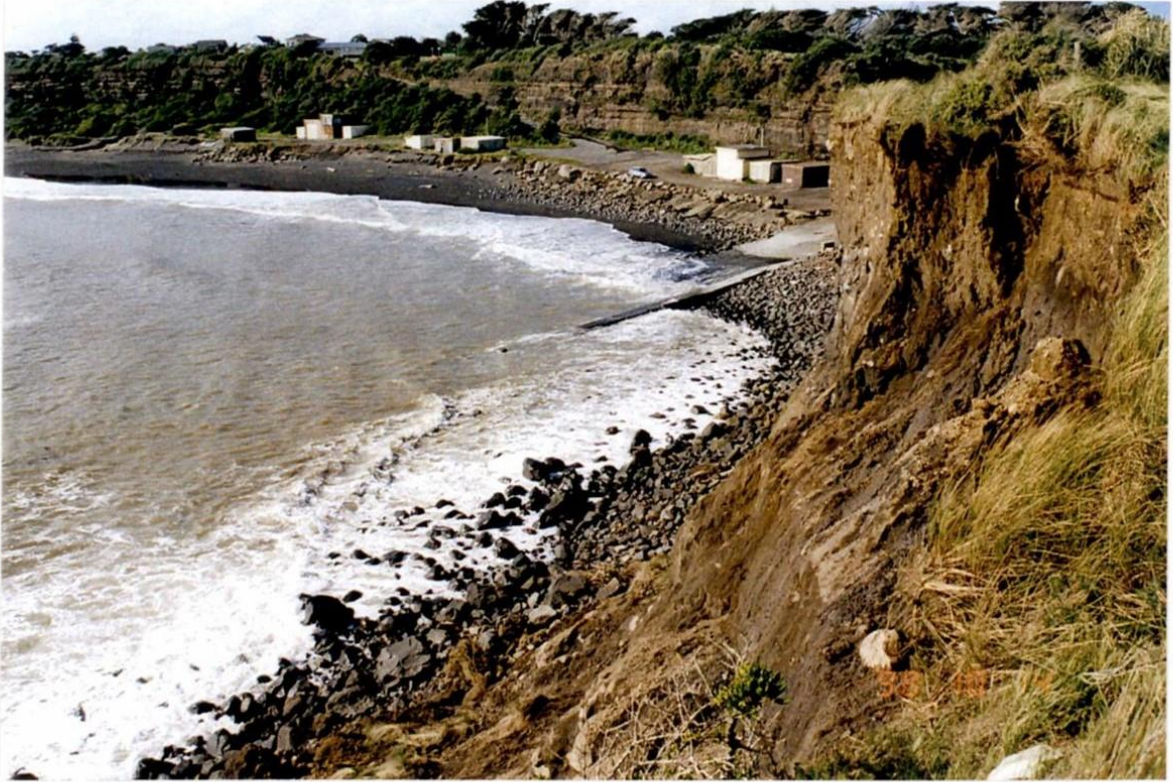
Figure 2: Recent landslip SW of the boat ramp and boulder beach providing some protection to the seacliffs from sea erosion (Photo: 14 October 1998).
