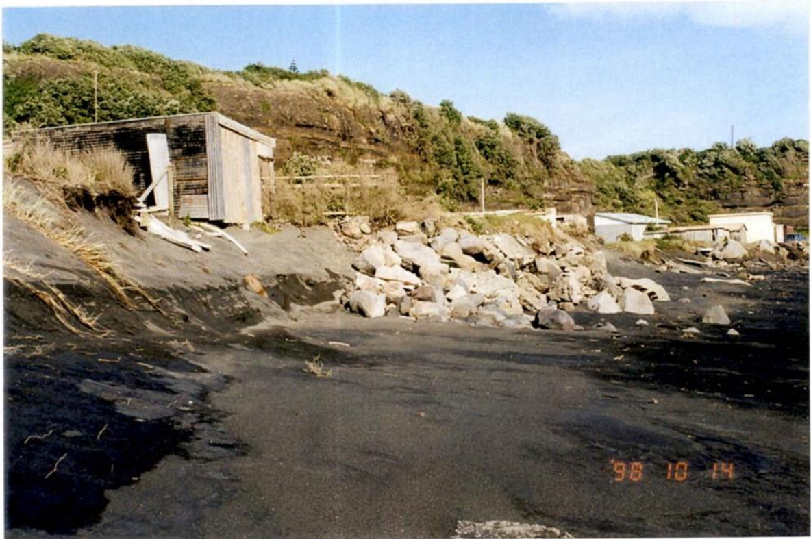
Figure 7: View SE showing the 20m-long rubble revetment which has caused up to 5m outflanking and the undermining of the 2 old boatsheds (Photo: 14 October 1998).
