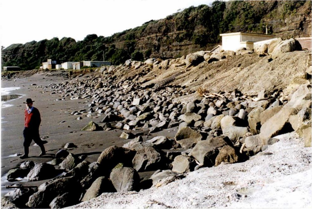
Figure 6: View NW from boat ramp showing the 80m-long concrete and rubble revetment overlying the natural boulder beach (Photo: 14 October 1998).
