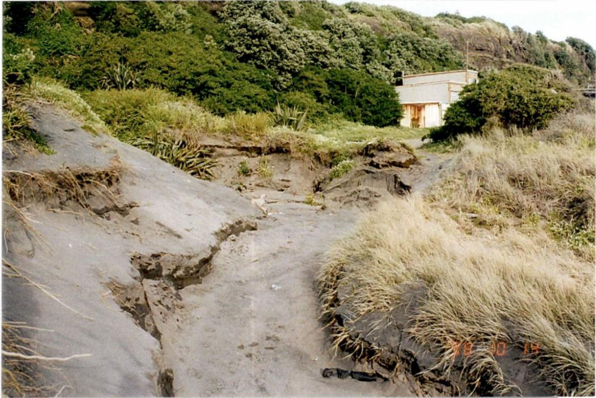
Figure 8: Washout in foredune complex from storm water discharging over the seacliffs behind (Photo: 14 October 1998).
