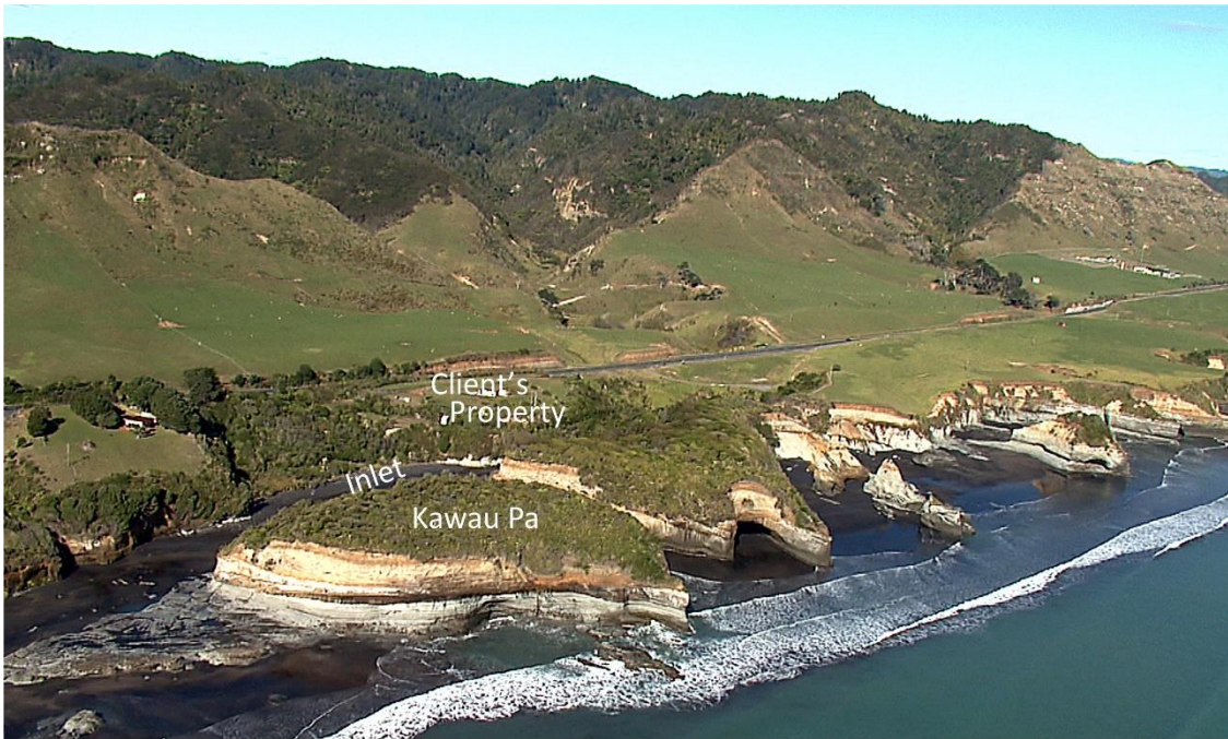
Figure 4 The open coast fronting the Middleton/Post property and the inlet. Caves, stacks and intertidal rock platforms attest to ongoing sequential and cyclic landscape change.
