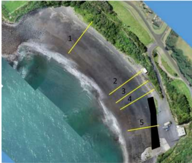
Figure 1 Middleton Bay where transects 1,2 and 5 are used for environmental monitoring and the additional transects 3 and 4 are required to identify any adverse effects from future modification (repair, strengthening) of the revetment structure – the existing structure is shown in black.
