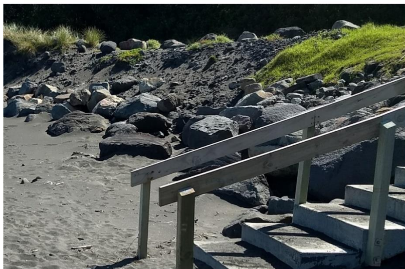
Figure 2.5 As-built photo taken 16-3-2020 (top) showing steps and newly place stone with battered bank (dune) in foreground. Lower photo taken 17 February 2022 showing stairs and area immediately northwest indicating past erosion. This area was identified by BECA as in urgent need of armour rock. It is also this area was designated to have a “return” build in to avoid future outflanking. Photos CSL
