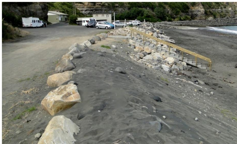
Figure 2.5 As-built photo taken 16-3-2020 (top) showing steps and newly place stone with battered bank (dune) in foreground. Lower photo taken 17 February 2022 showing stairs and area immediately northwest indicating past erosion. This area was identified by BECA as in urgent need of armour rock. It is also this area was designated to have a “return” build in to avoid future outflanking. Photos CSL
