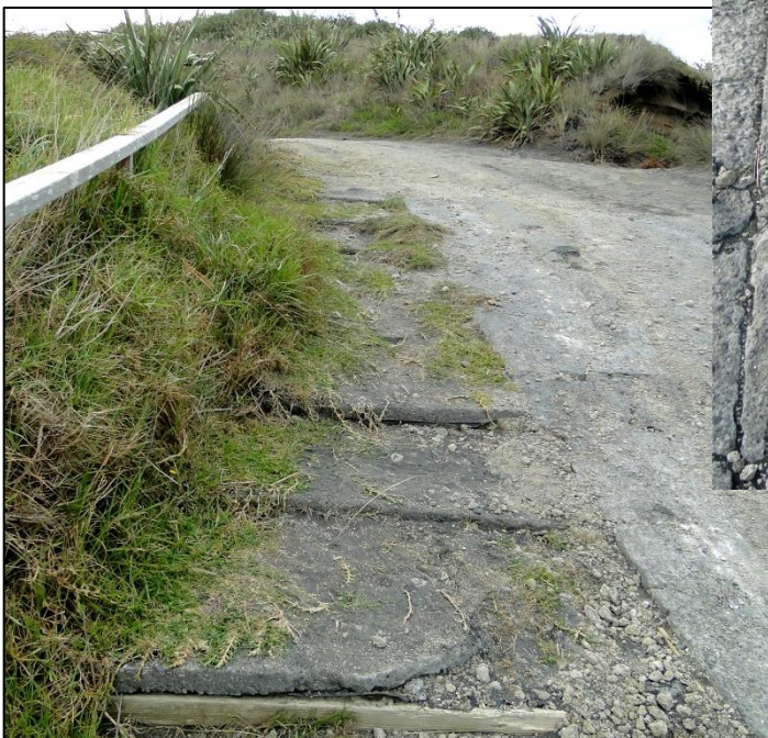
Figure 6.4 Dysfunctional access steps and handrail, with fine shell rock coating the ramp and steps.
