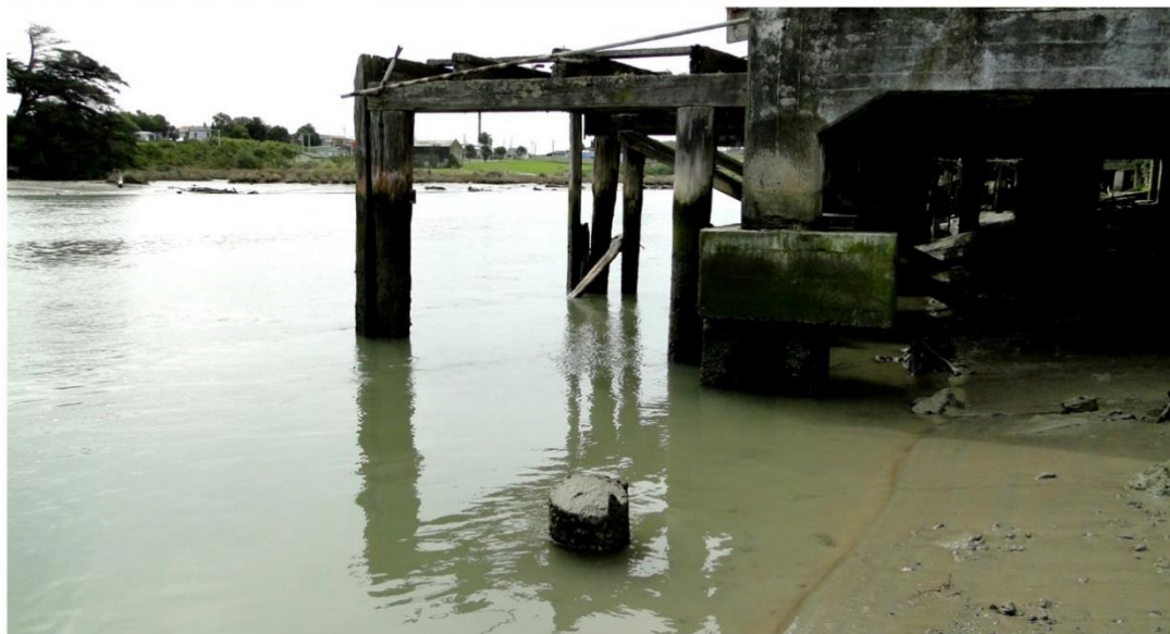
Figure 5.4 Upper photo: piles in the vicinity of the wharf buildings - between 420 to 465 m. Middle photo: superstructure fronting the wharf buildings at about 500 m chainage. Lower photo: downstream end of wharf (530 m).
