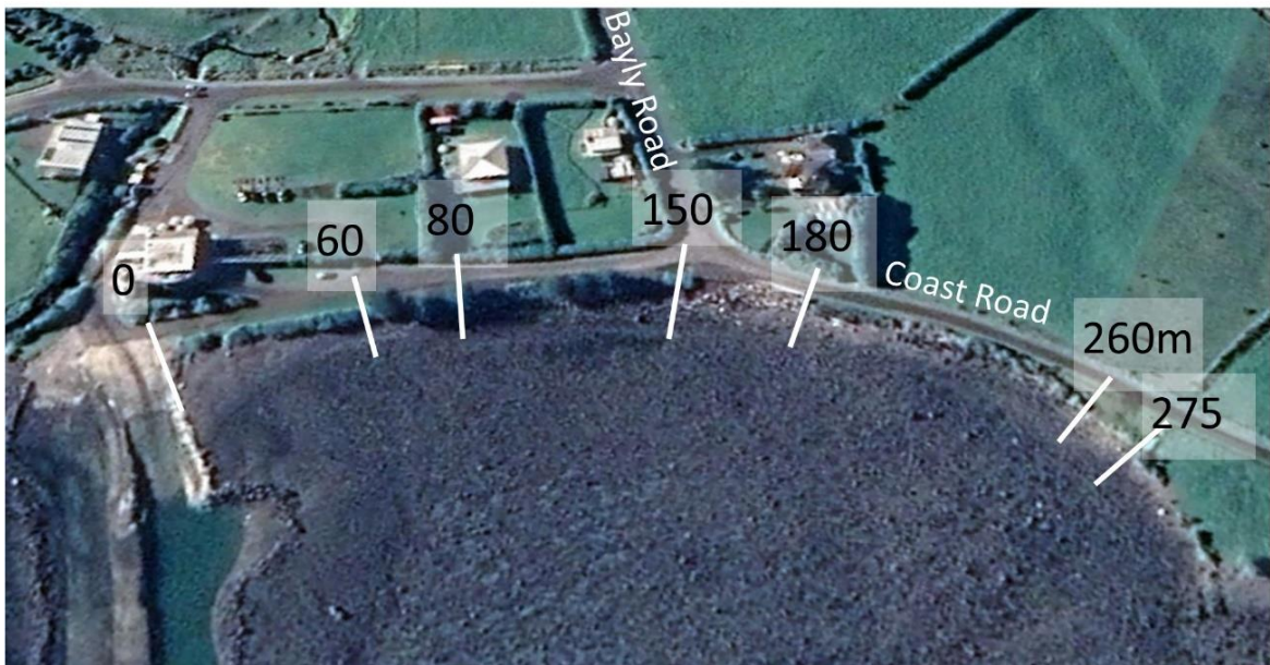
Figure 2.2 Bayly Road seawall location with chainage marked from the boat launching structure.
