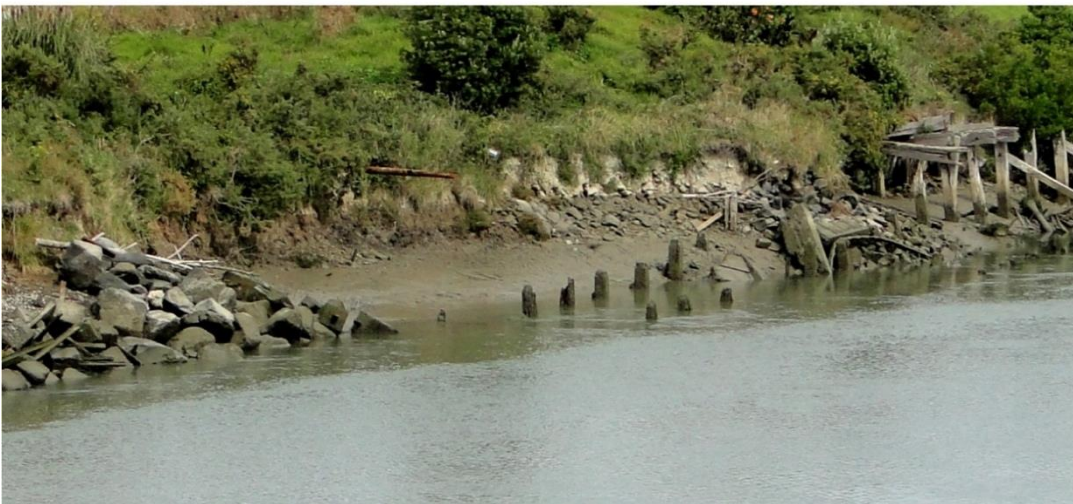
Figure 5.2 Upper photo: Rip-rap near the bridge comprising variety of materials with no coverage in places. Middle photo: more complete rip-rap protection but hazardous iron rails in distance. Lower photo: variable riprap at the rip-rap/wharf juncture.
