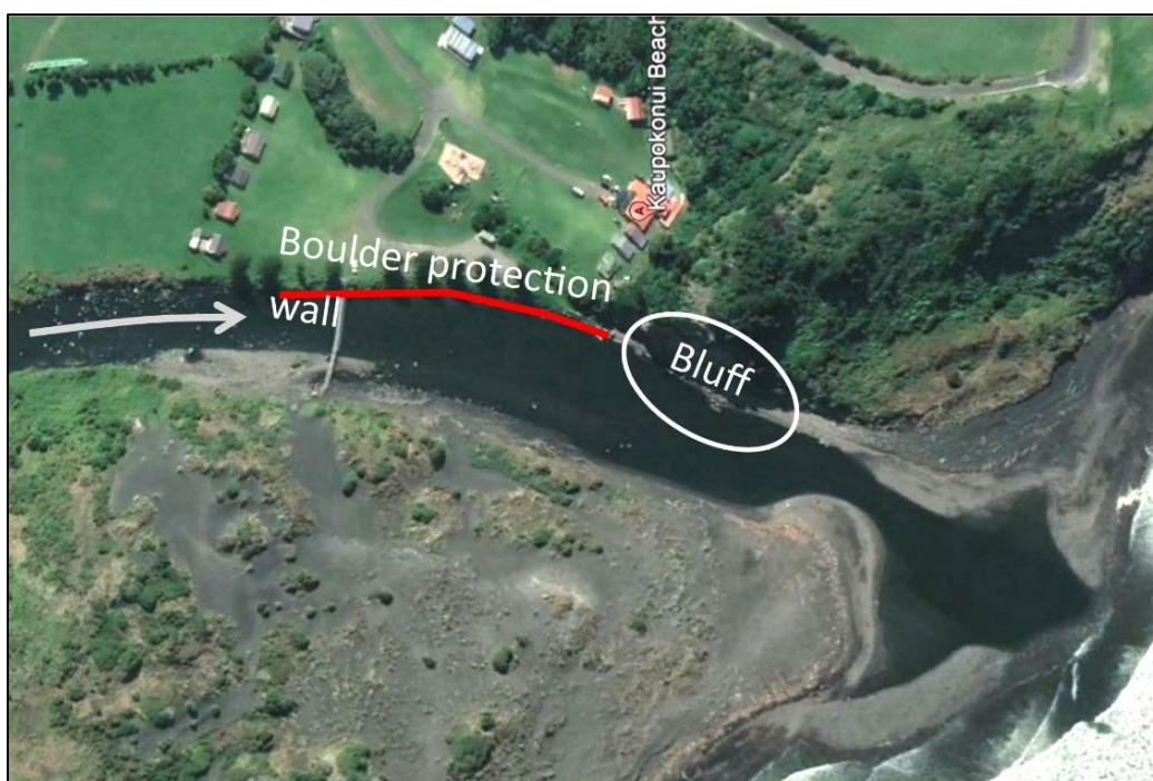
Figure 3.1 Location of the 170 m long boulder protection wall, the eastern bluff (Kaupokonui South Head), and footbridge (evident but not marked). The arrow indicates river flow and the beach is on the right.
