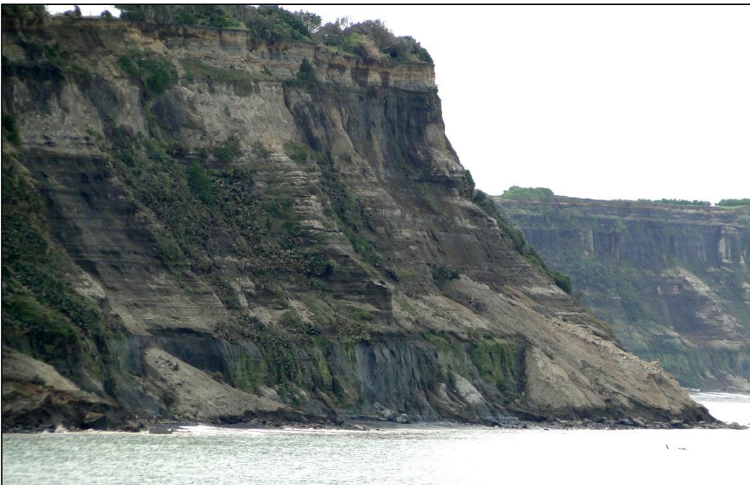
Figure 4.3 Recent coastal cliff erosion and debris spilling across the beach between Waihi and Ohawe Beaches.
