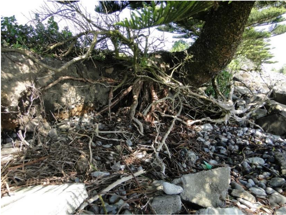
Figure 2.4 Typical upper bank exposure and undermined Norfolk pine trees at 60 to 80 m chainage.
