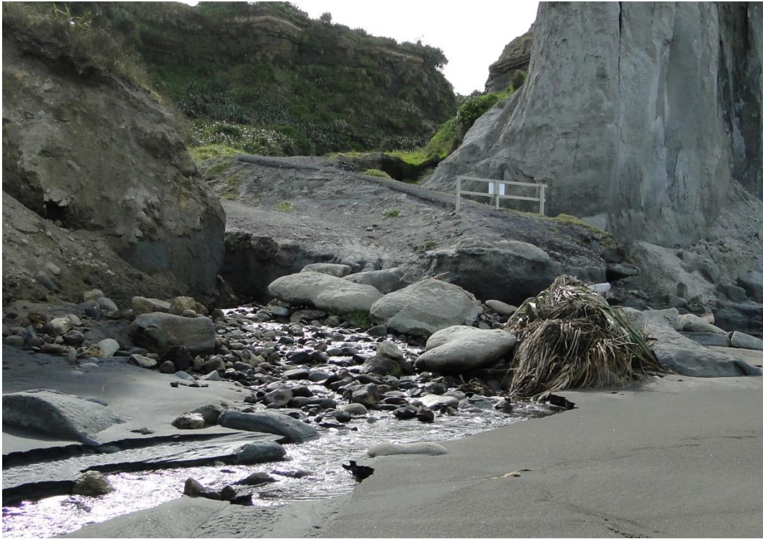
Figure 4.2 The barrier marks the location of the original consented gabion-based access structure. The alternative lower accessway (from 2018) is evident as is the escarpment at its base caused by stream flow and waves. Boulder-hopping is now required to access the beach.
