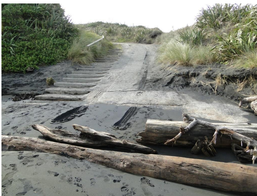
Figure 6.1 Caves beach access structure, showing pedestrian steps and handrail, vehicle ramp and broadened lower section.
