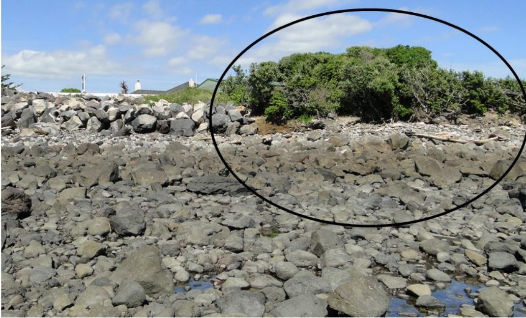
Figure 2.7 Exposed upper bank (circled) at southern end of the recent rock placement on the left side of photo (180 to 200 m chainage).
