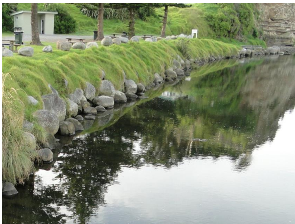
Figure 3.2 Kaupokonui boulder protection wall post flood with bluff in background.
