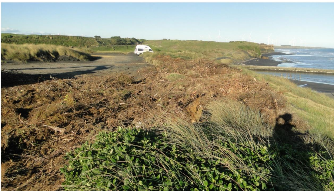
Figure 9 Green waste placement made on 29-4-2022 at Site D. The top photo shows green waste filling the gut at the dune crest filled with green waste, while the lower photo shows green waste infilling the landward erosion area illustrated in Figure 3.
