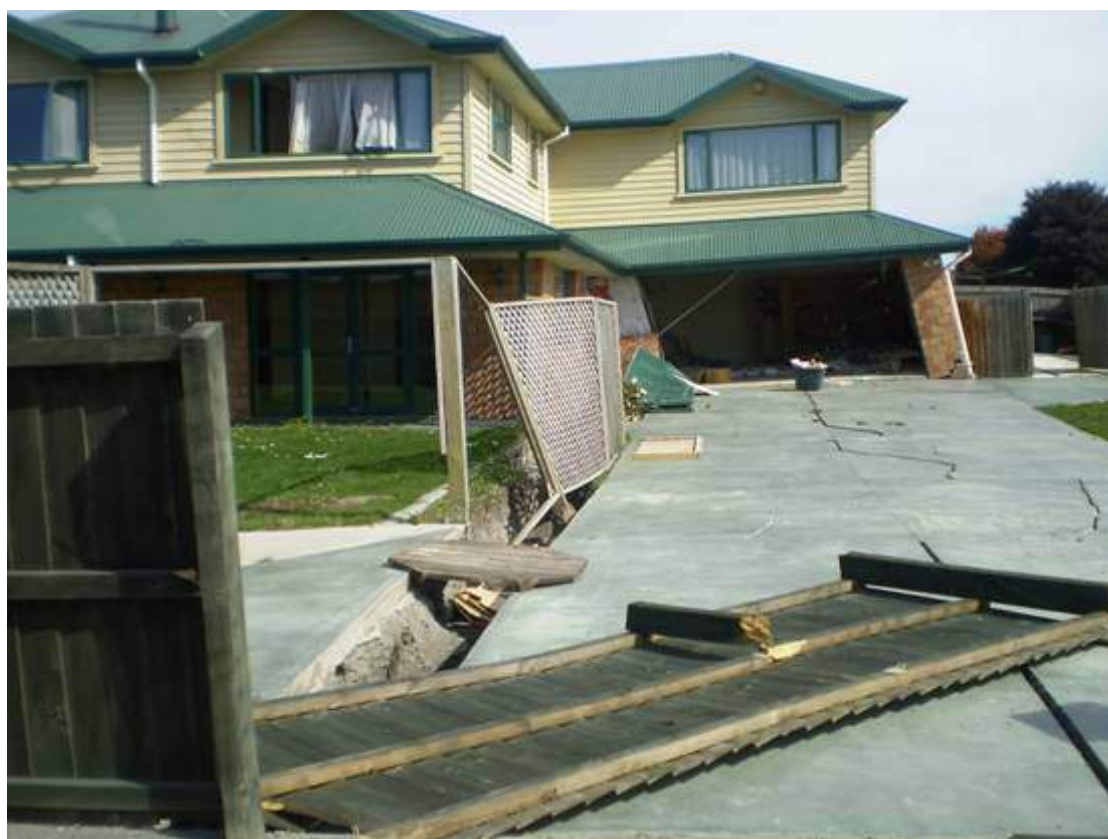
Figure 2.7 Liquefaction-induced lateral spreading through the foundation of a house in Kaiapoi approximately 45 kilometres from the epicentre of the magnitude 7.1, 4 September 2010 Darfield earthquake. (Photo: Tonkin + Taylor Ltd).
