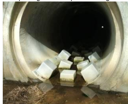
Figure 11-7 Culvert with Energy Dissipation Baffles
