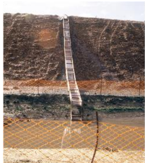
Figure 8-13 Flume to a sediment retention pond
