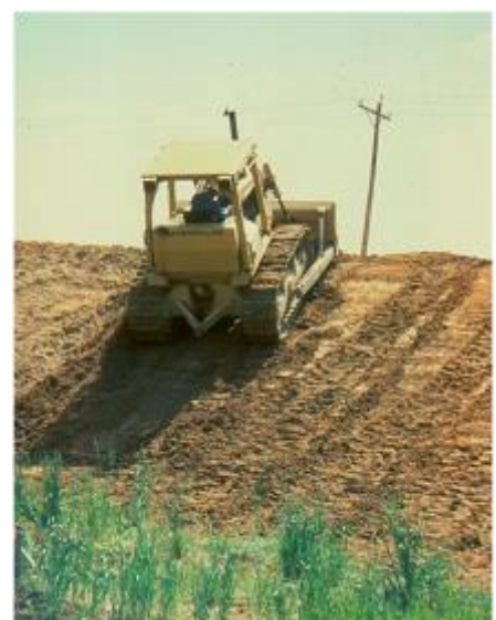
Figure 8-16 Surface roughening with a bulldozer
