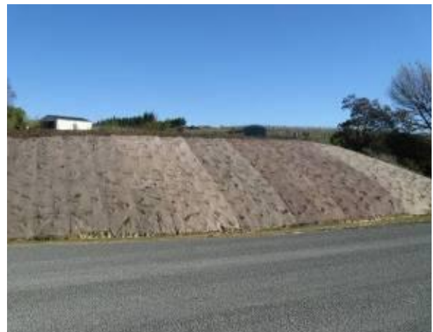
Figure 8-36 Plastic cover providing slope protection with plantings placed throughout the cover
