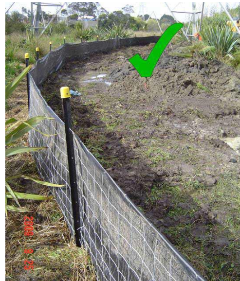
Figure 9-14 Super Silt Fence
