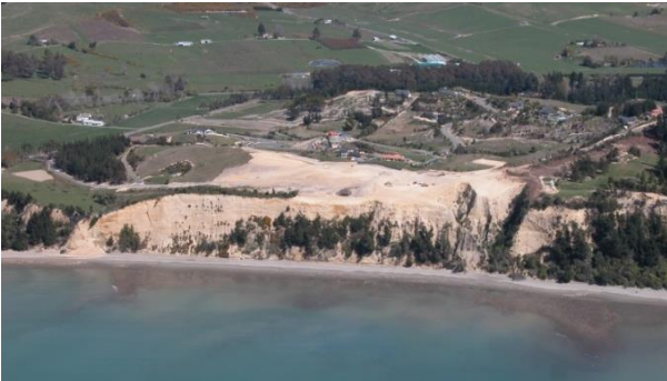
Figure 4-14 Visual impact of land disturbance
