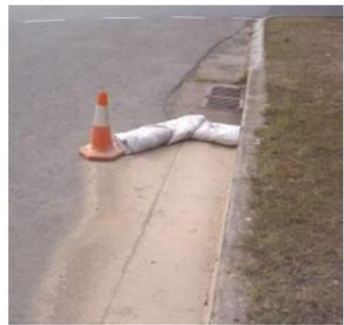
Figure 9-27 Sandbag check dam in gutter
