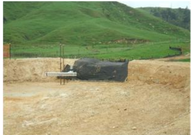
Figure 9-16 Decanting Earth Bund
