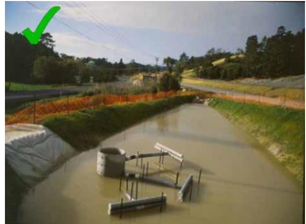
Figure 9-5 Sediment retention pond detail showing multiple decants
