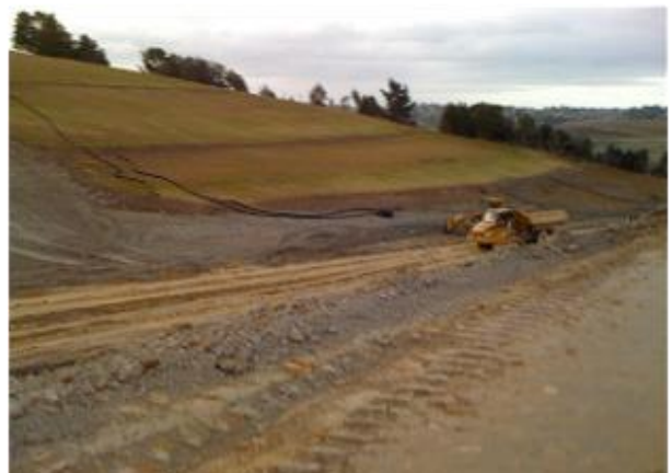
Figure 8-5 Contour drains established on embankments as a water control measure in conjunction with progressive stabilisation.
