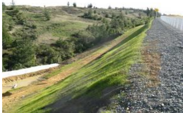
Figure 6-8 Road Construction with Slope Revegetation
