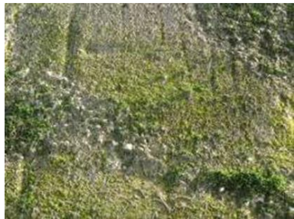
Figure 8-247 Recently applied hydroseed showing emergent grass growth
