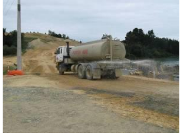
Figure 8-39 Dust suppression by water sprinkling
