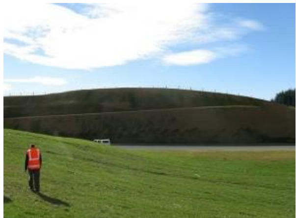
Figure 8-21 Vegetative stabilisation is an effective erosion control practice
