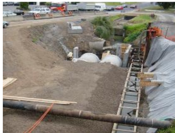
Figure 11-15 Use of Marine Ply flume as a Stream Diversion
