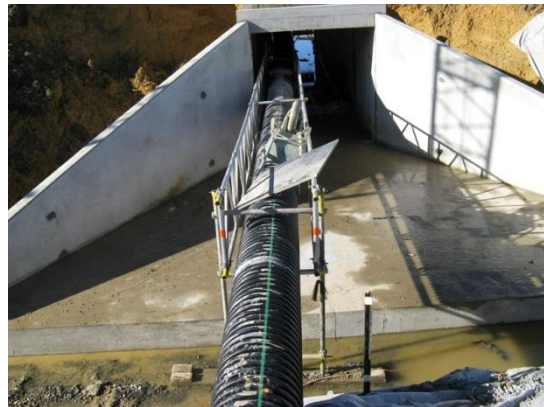
Figure 11-13 Pipe diversion during Ruby Bay Bypass (D.Shaw)
