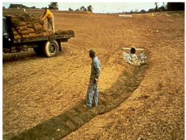
Figure 8-3326 Turf being applied for a swale outfall
