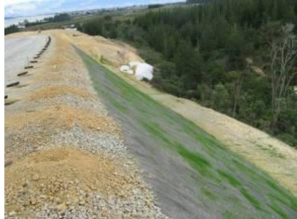
Figure 8-34 Erosion control blanket for slope protection. Notice grass growing through blanket
