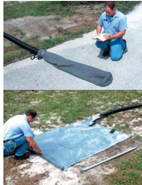
Figure 9-22 Dewatering Pipe Sock and Bag
