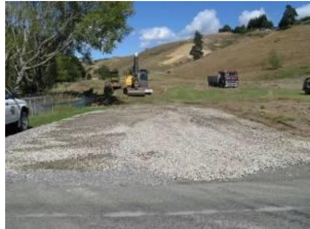
Figure 8-20 Stabilised Entraceways
