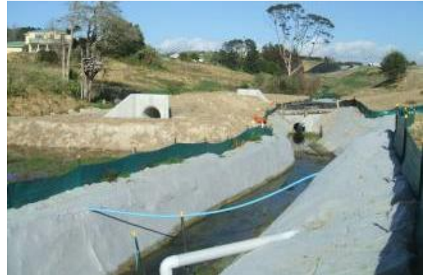
Figure 11-20 Temporary diversion and culvert while a new permanent culvert is constructed
