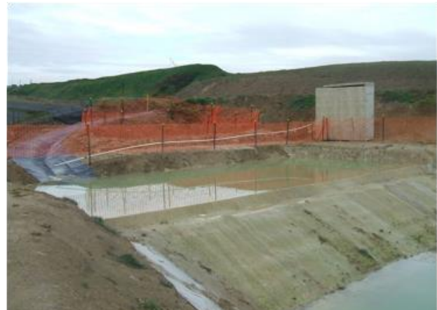
Figure 9-3 Level Spreader and Forebay
