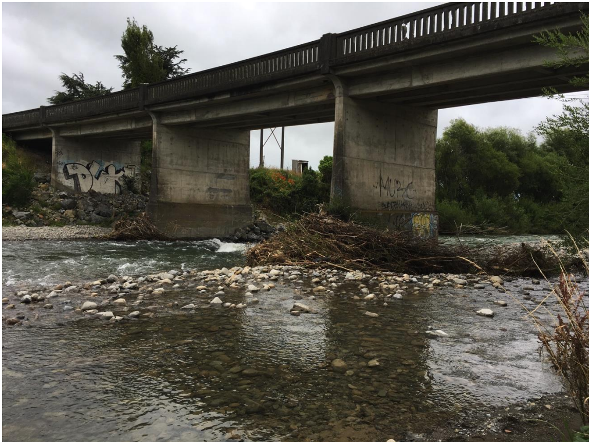
Figure 27: Ōhau River and Bridge
