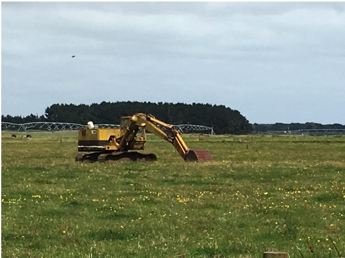
Figure 16: Digger in the middle of a paddock used to clear drains
